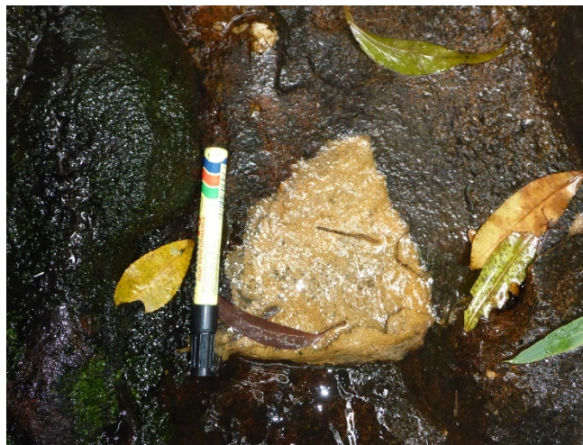
Photo 4: DA3B_LW13_046 , looking at the section of rock displacement. Taken 01/04/2019.
