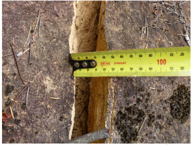
Photo 6: DA3B_LW14_019, looking at the width of the fracturing. Taken 20/02/2019.
