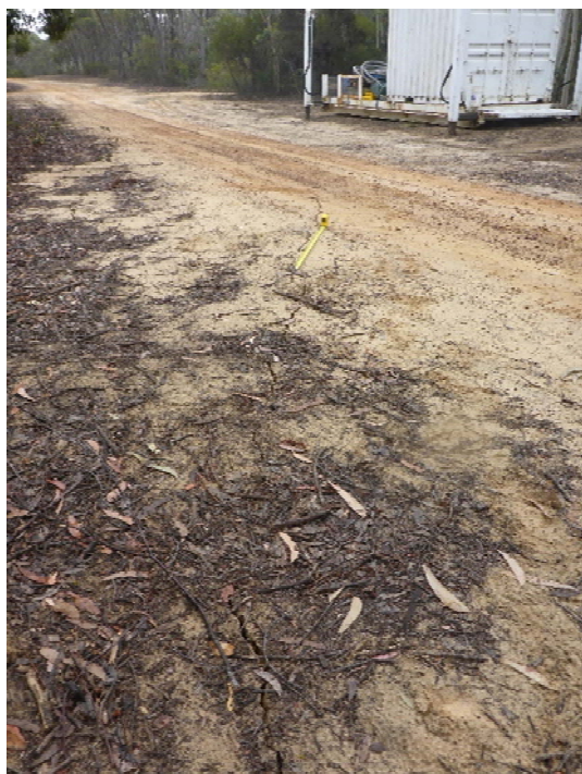
Photo 1: Impact DA3B_LW14_009. Taken on 03/09/18.
