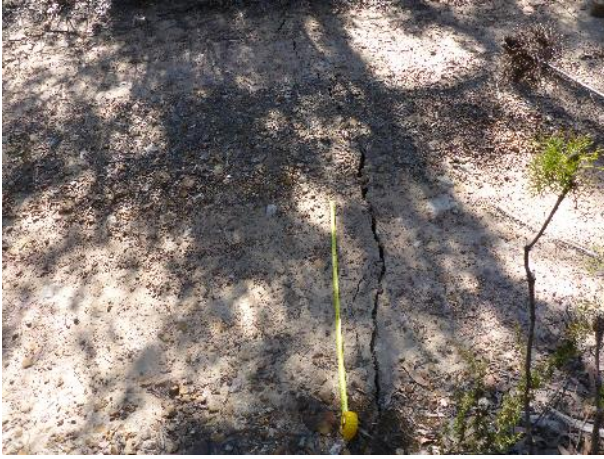
Photo 3: Impact DA3b_LW14_003. Taken on 7/07/18.
