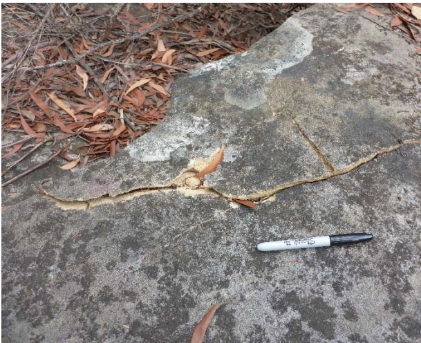
Photo 9: DA3B_LW14_022, looking at the rock fracturing. Taken 20/02/2019.
