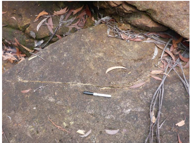
Photo 12: DA3B_LW14_021 , looking at the section of rock fracturing. Taken 20/02/2019.
