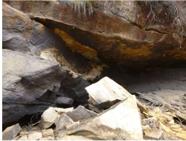
Photo 6: DA3B_LW14_015, looking at the rockfall. Taken on 6 December 2018.
