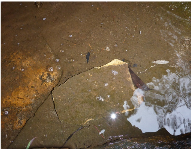
Photo 7: DA3B_LW13_042, looking at a section of new rock fracturing. Taken 01/04/2019.
