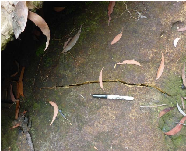
Photo 11: DA3B_LW14_021 , looking at the section of rock fracturing. Taken 20/02/2019.
