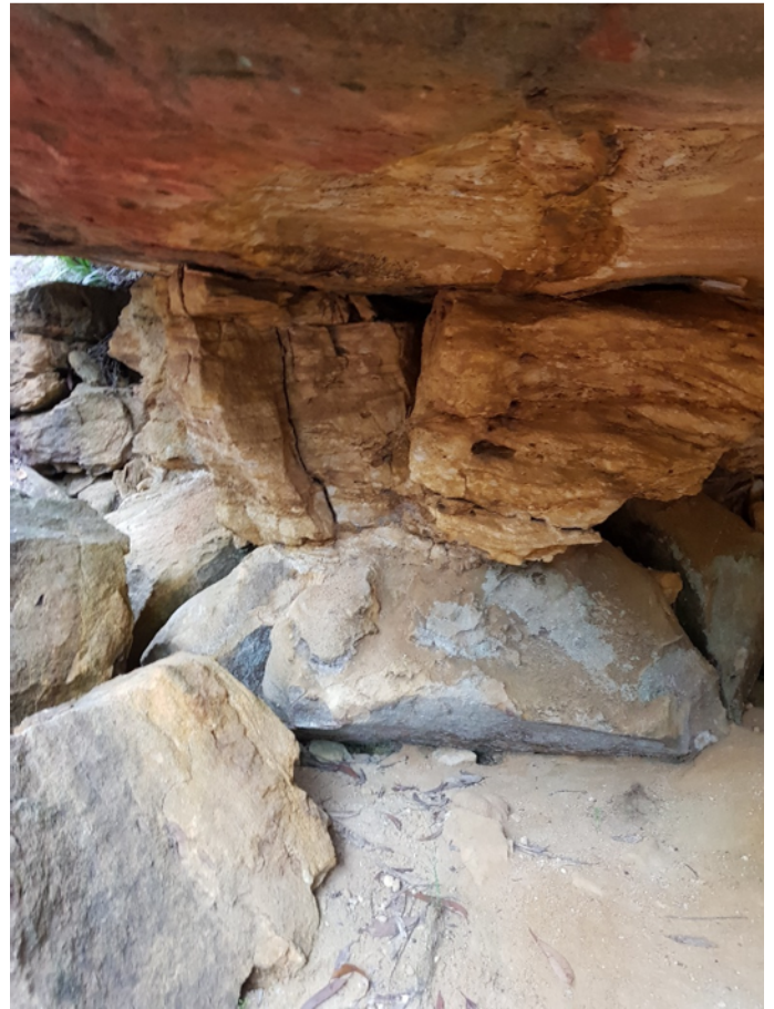
Photo 5: DA3B_LW14_027, looking at a section of rock fracturing. Taken 10/05/2019.
