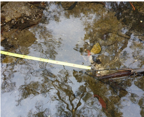
Photo 1: DA3B_LW14_023 , looking at a section of rock fracturing. Taken 01/04/2019.
