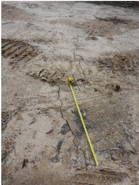
Photo 7: Impact DA3B_LW14_007. Taken on 28/08/18.
