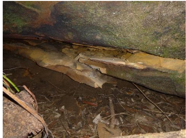
Photo 6: Impact DA3b_LW13_044. Taken on 26/07/18.
