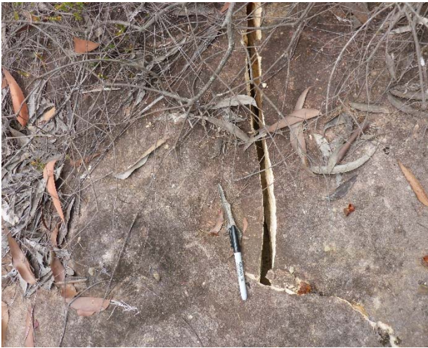
Photo 7: DA3B_LW14_019, looking at a section of rock fracturing. Taken 20/02/2019.
