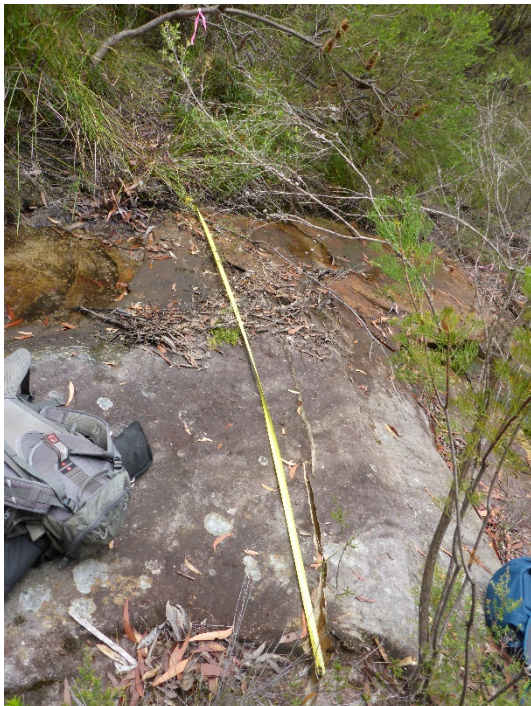
Photo 5: Fracturing across rockbar. Taken on 21/01/2019.
