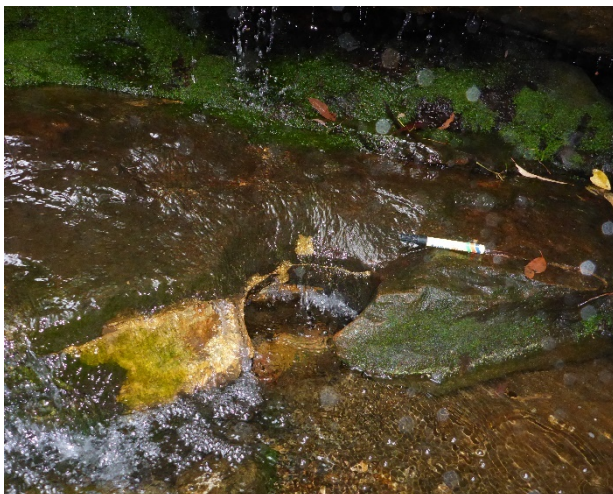
Photo 3: DA3B_LW13_046 , looking at the extent of the rock fracturing. Taken 01/04/2019.
