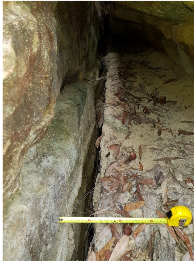
Photo 3: DA3B_LW14_026, looking at a section of displacement. Taken 10/05/2019.
