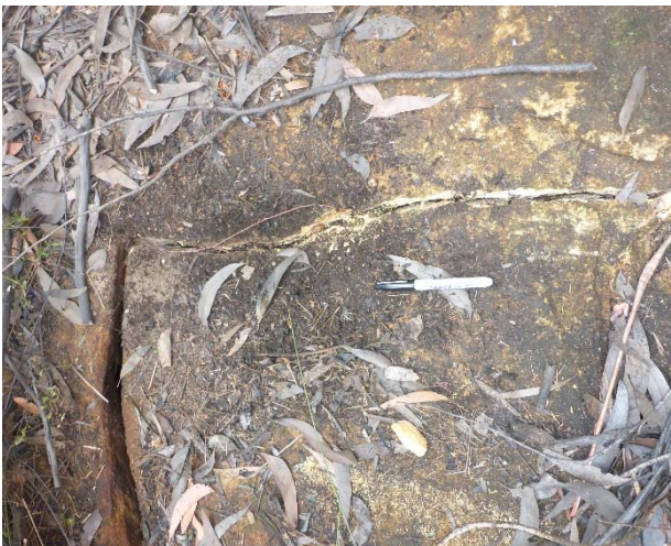
Photo 3: DA3B_LW14_018, looking at the extent of the rock fracturing. Taken 20/02/2019.
