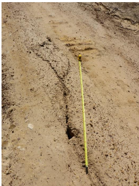
Photo 1: Impact DA3B_LW14_010. Taken on 10/09/18.
