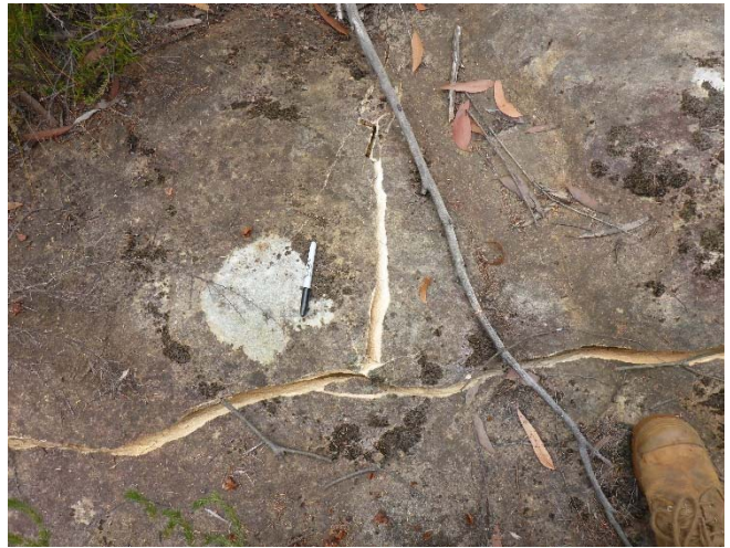
Photo 8: DA3B_LW14_019, looking at a section of rock fracturing. Taken 20/02/2019.
