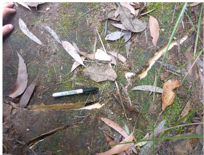
Photo 2: DA3B_LW14_017 , looking at a section of rock fracturing. Taken 20/02/2019.
