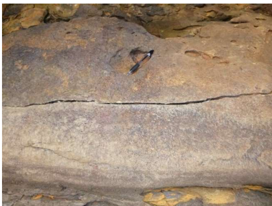
Photo 1: DA3B_LW13_043, looking at a section of rock fracturing. Taken on 6 December 2018.
