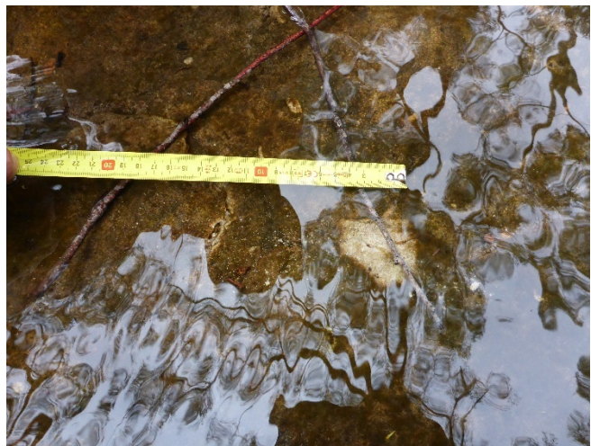
Photo 2: DA3B_LW14_023 , looking at a section of rock fracturing. Taken 01/04/2019.
