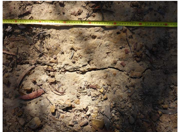
Photo 6: Impact DA3B_LW14_006. Taken on 19/08/18.
