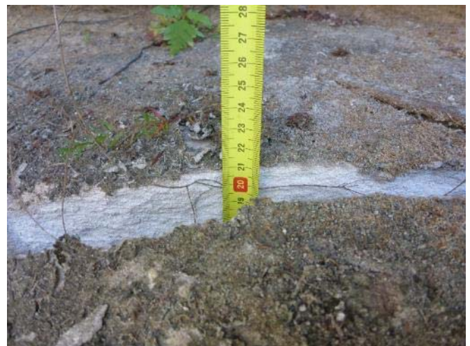
Photo 2: DA3B_LW14_024 , looking at the depth of rock fracturing. Taken 09/04/2019.
