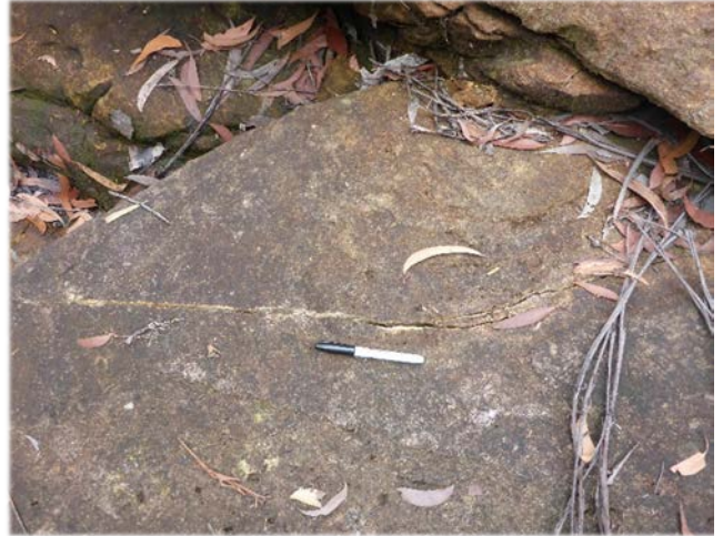
Photo 24: DA3B_LW14_021, looking at the section of rock fracturing. Taken 20/02/2019.
