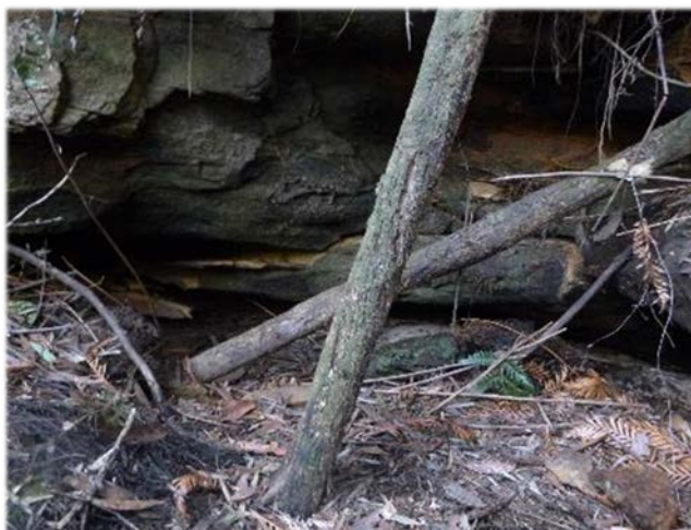
Photo 5: DA3b_LW13_044 , looking at a section of rock fracturing. Taken 26/07/18.
