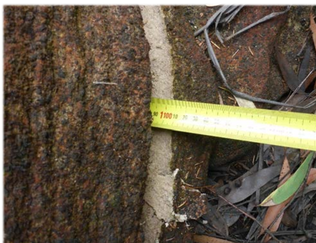
Photo 22: DA3B_LW14_020, looking at the depth of the fracturing. Taken 20/02/2019.
