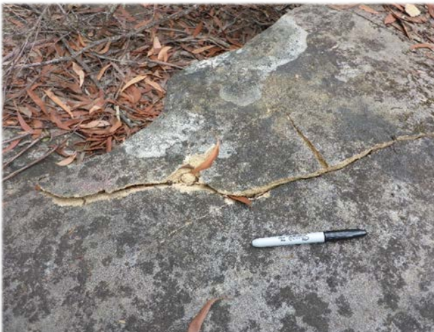
Photo 25: DA3B_LW14_022, looking at the section of rock fracturing. Taken 20/02/2019.
