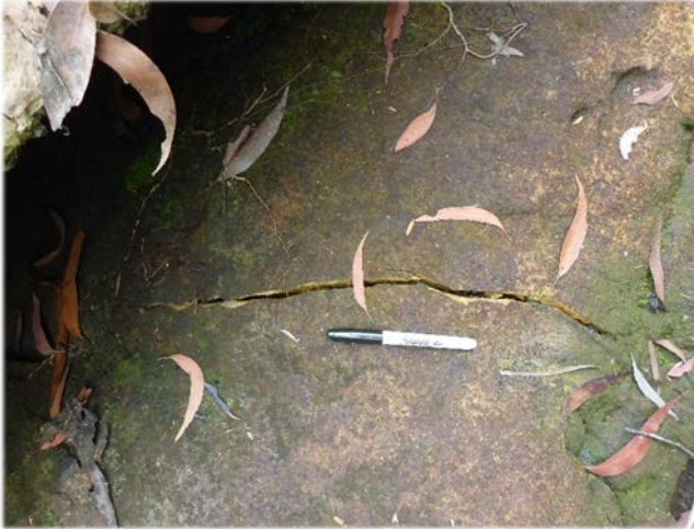
Photo 23: DA3B_LW14_021, looking at the section of rock fracturing. Taken 20/02/2019.
