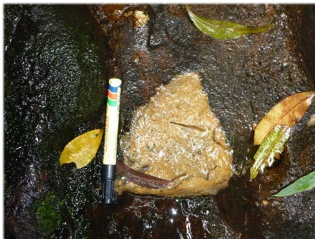
Photo 12: DA3B_LW13_046, looking at the section of rock displacement. Taken 01/04/2019.
