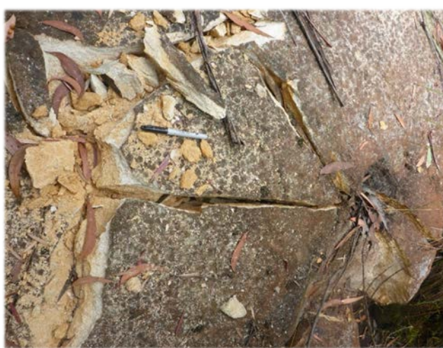
Photo 14: DA3B_LW14_016, looking at fracturing and dislodged sections of rock. Taken on 21/01/2019.
