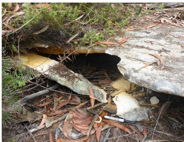
Photo 13: DA3B_LW14_016, looking at fracturing and dislodged rock segments. Taken on 21/01/2019.
