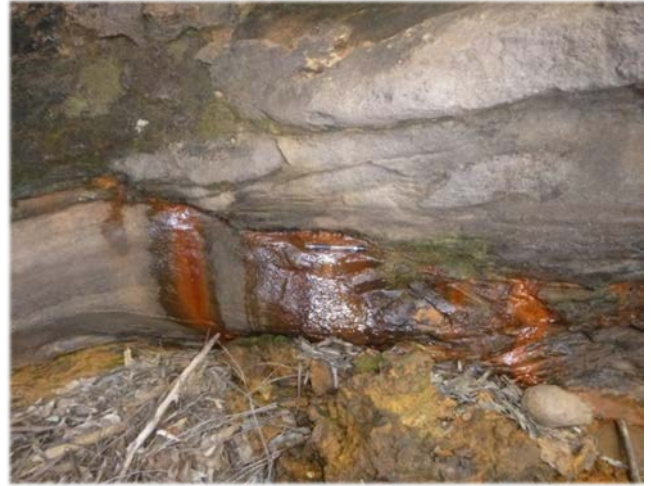
Photo 8: DA3B_LW13_043, looking at iron staining. Taken 6/12/2018.
