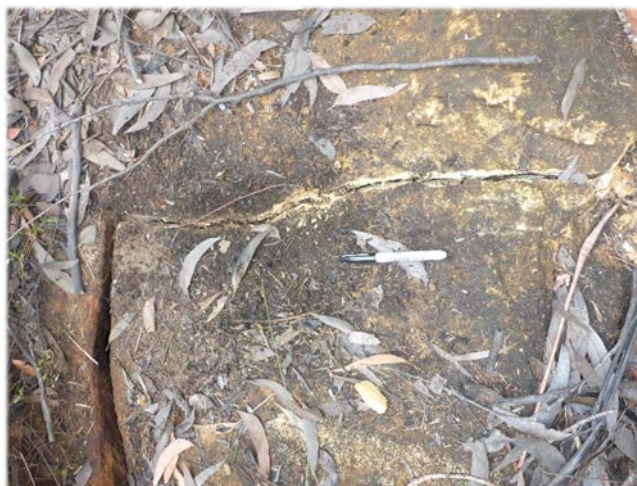
Photo 17: DA3B_LW14_018, looking at the extent of the rock fracturing. Taken 20/02/2019.
