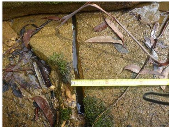
Photo 10: DA3b_LW13_045, Looking at the rock fracturing. Taken 8/07/18.
