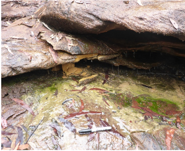
Photo 29: DA3B_LW13_035, fracturing with flow diversion across small step on rockbar. Taken on 21/01/2019.
