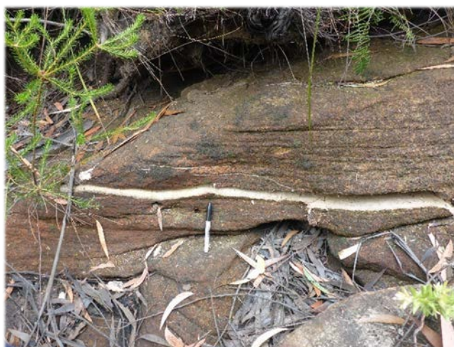
Photo 21: DA3B_LW14_020, looking at the extent of the rock fracturing. Taken 20/02/2019.
