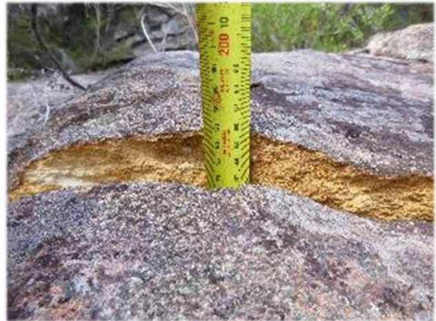
Photo 18: DA3B_LW13_023, closeup of the deepest section of fracturing. Taken 29 th March 2018.
