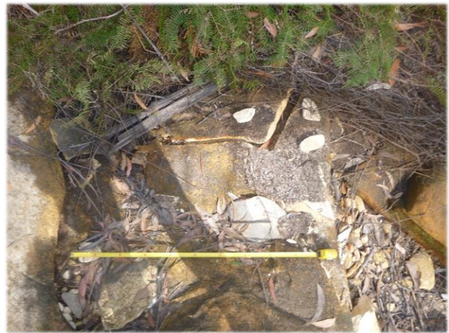
Photo 37: Impact DA3B_LW13_006 , looking across pool at fracturing. Taken on 3/10/2017.
