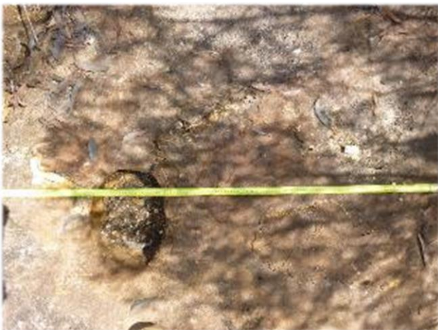
Photo 9: DA3B_LW13_021, looking at the small section of plating. Taken 29 th March 2018.
