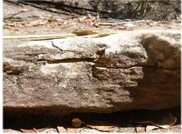
Photo 20: DA3B_LW13_028, looking upstream at largest section of fracturing. Taken 5 th April 2018.
