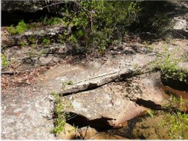
Photo 19: DA3B_LW13_028, looking upstream at the extent of the impact. Taken 5 th April 2018.
