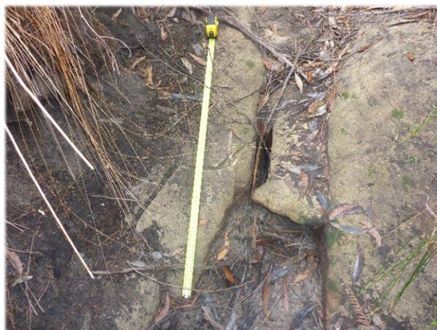
Photo 41: Impact DA3B_LW13_009 , looking upstream, taken on 23/10/2017.
