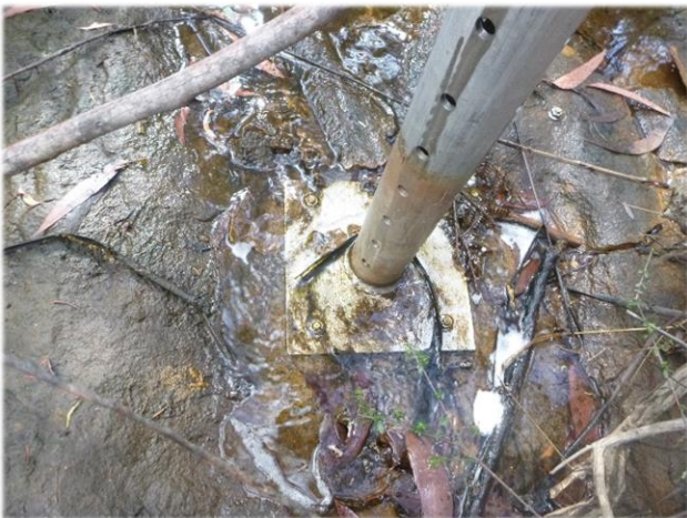
Photo 3: Flow diversion adjacent to monitoring equipment at LA4S1. Taken on 3 rd May 2017.
