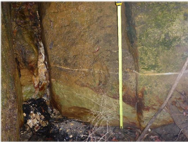
Photo 42: Impact DA3B_LW13_010 looking upstream, taken 27/10/2017.
