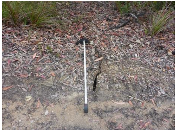
Photo 2: DA3B_LW12_020 - Soil cracks on access track. Taken on 15/11/2016
