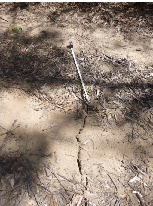
Photo 3: DA3B_LW12_017 – Soil cracking across AT6AA. Taken on 9/11/2017
