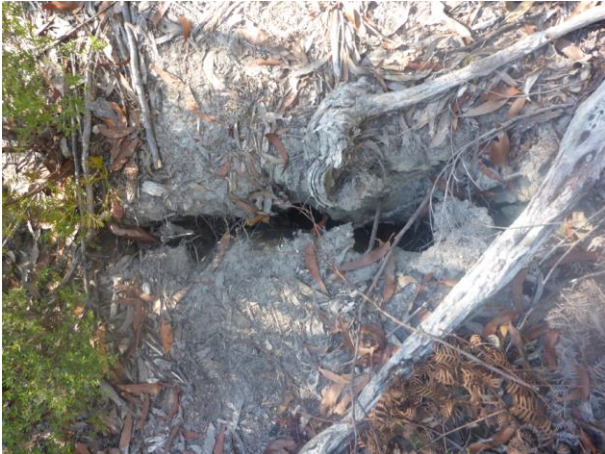
Photo 5: DA3B_LW12_025 –Soil cracking across access track. Taken on 18/05/2017
