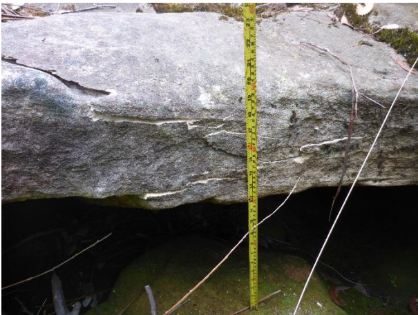
Photo 9: DA3B_LW12_019 – Fracturing to the face of a step in WC21_Step 48. Taken on 9/11/2016.
