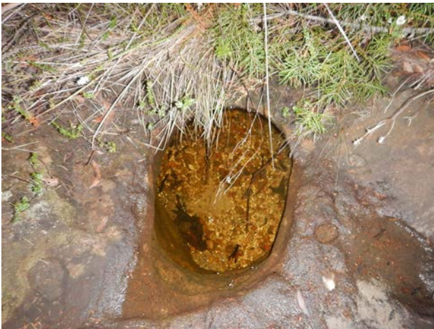
Plate 6 WC21 Pothole B
