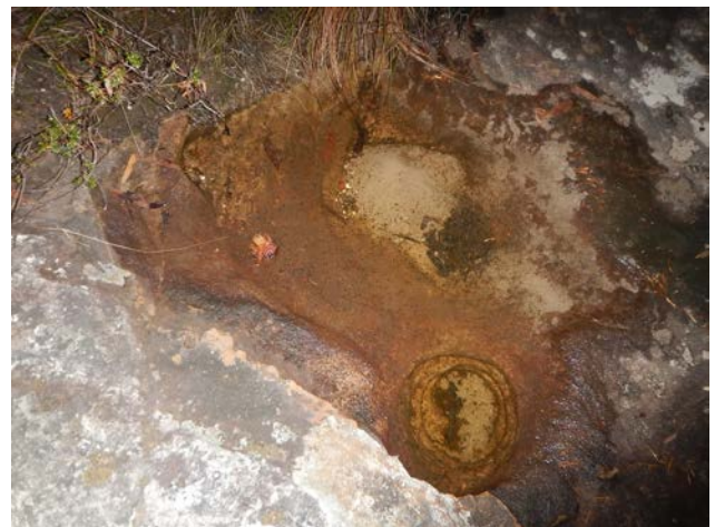
Plate 9 WC21 Pothole E
