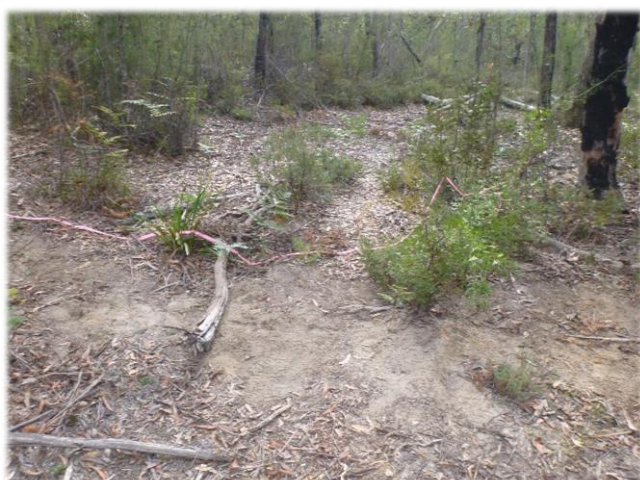
Photo 26: DA3B_LW12_025 -Section of remediated cracking across access track. Taken on 18/05/2017.
