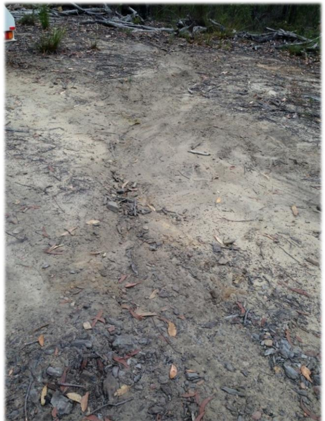
Photo 23: Remediation of DA3B_LW12_017. Taken on 18/01/2017.
