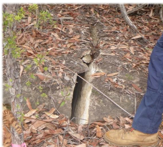
Photo 25: DA3B_LW12_025 -Rock fracture extending from access track. Taken on 20/01/2017.
