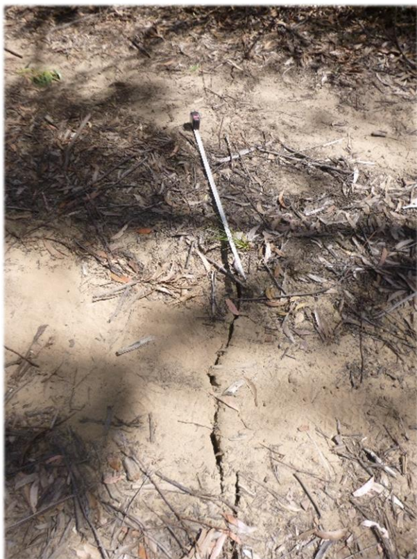
Photo 18: DA3B_LW12_017 – Soil cracking across AT6AA. Taken on 11/10/2016.
