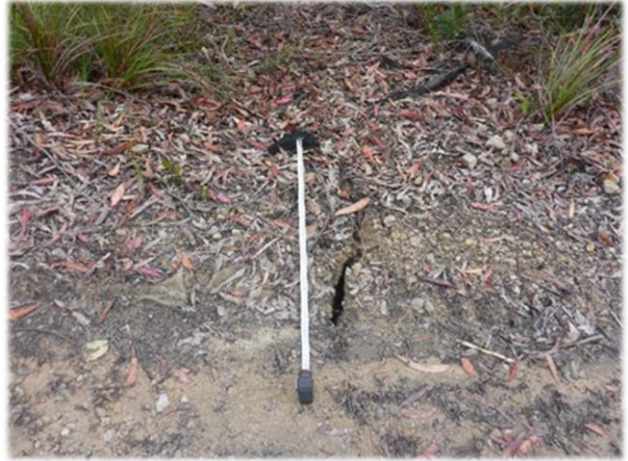
Photo 21: DA3B_LW12_020 - Soil cracks on access track. Taken on 15/11/2016.
