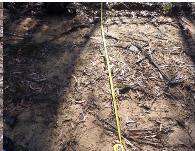
Photo 10: DA3B_LW11_005- Soil crack, looking along seismic track. Taken on 19/09/15.
