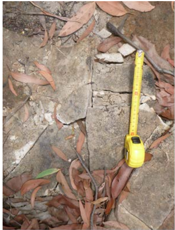
Photo 6: DA3B_LW11_008- Rock fracture, looking along WC21. Taken on 14/01/2016.
