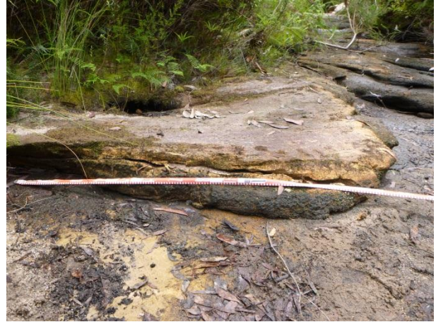
Photo 7: Impact DA3b_LW10_011 – Fracturing with dislodged fragment. Taken on 25/11/2014
