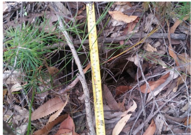
Photo 15: Impact DA3B_LW10_024. Width of crack. Taken on 18/02/2015
