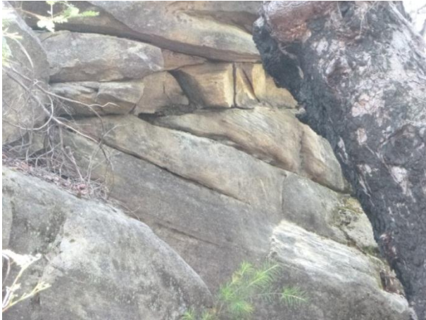
Photo 22: Impact DA3B_LW10_004 – Fracturing on cliff face. Taken on 27/10/2014
