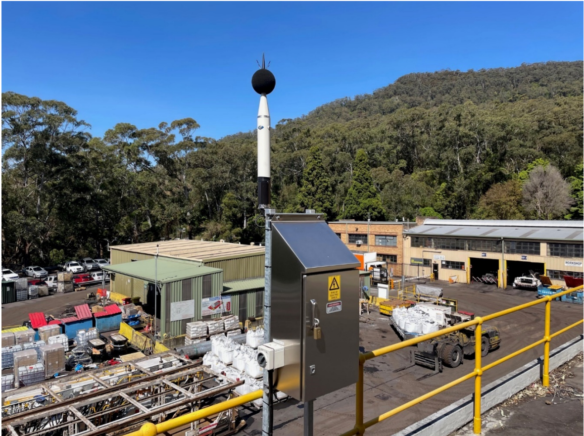
Plate 3: Real-time noise monitor on roof of Operations Building (Pit Top)
