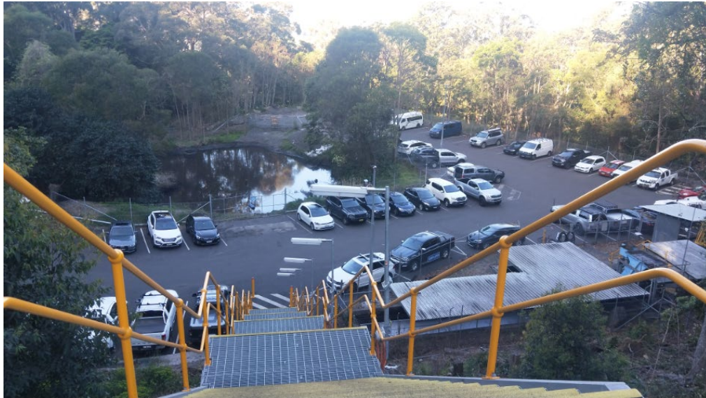
Plate 2: Sediment pond carpark and stairs to main parking area.
