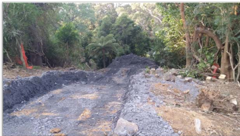
Figure 27: Fill material being delivered to site 23/6/2014
