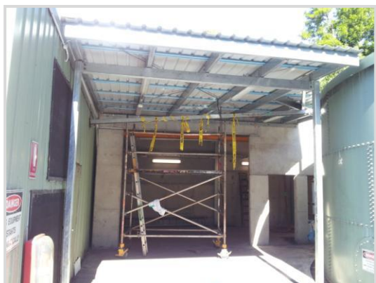
Figure 1: Construction of compressor building
