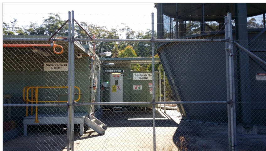
Figure 2: Tube bundle shed
