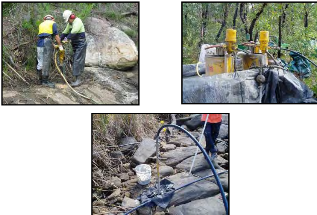
Figure 2-5: Rockbar Grouting in the Georges River
