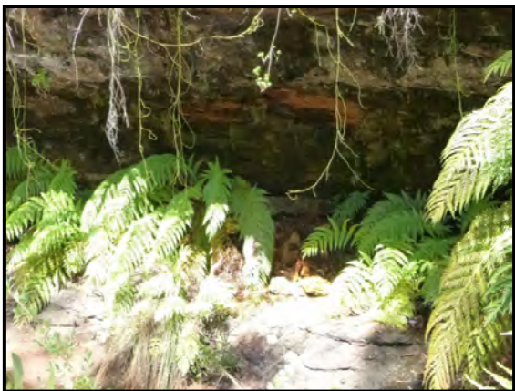
Photo 126: Impact LW9_027, small rockfall adjacent to Pool 10. Taken on 28 January 2014.
