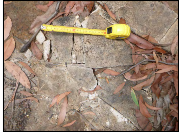
Photo 44: Impact LW11_008- Rock fracturing to upstream from WC21_Pool 30. Taken on 14 January 2016.
