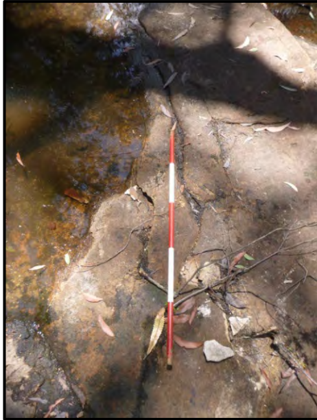
Photo 52: Impact LW11_010- Fracturing to Rockbar 27. Taken on 11 February 2016.
