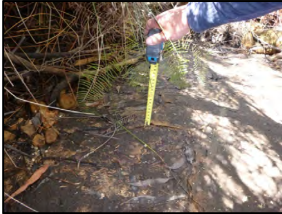
Photo 70: Impact LW10_008- fracturing and decline in surface flow, looking upstream. Taken on 25 November 2014.
