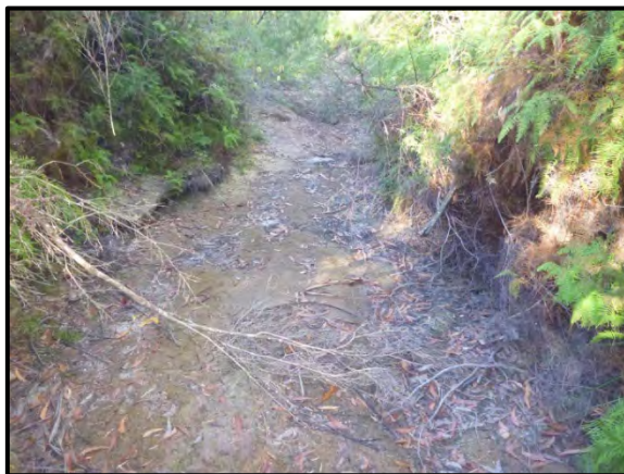
Photo 58: WC21_Rockbar 26, looking upstream. Taken on 23 March 2016.
