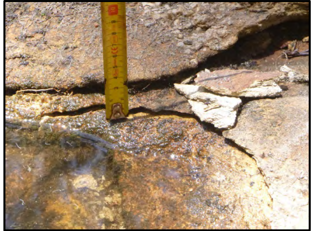
Photo 53: Impact LW11_010- Fracturing to Rockbar 27. Taken on 11 February 2016.
