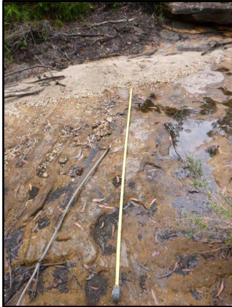
Photo 82: Impact DA3B_LW10_014- Fracture to base of WC21_Pool 23, looking across stream. Photo taken on 4 December 2014.
