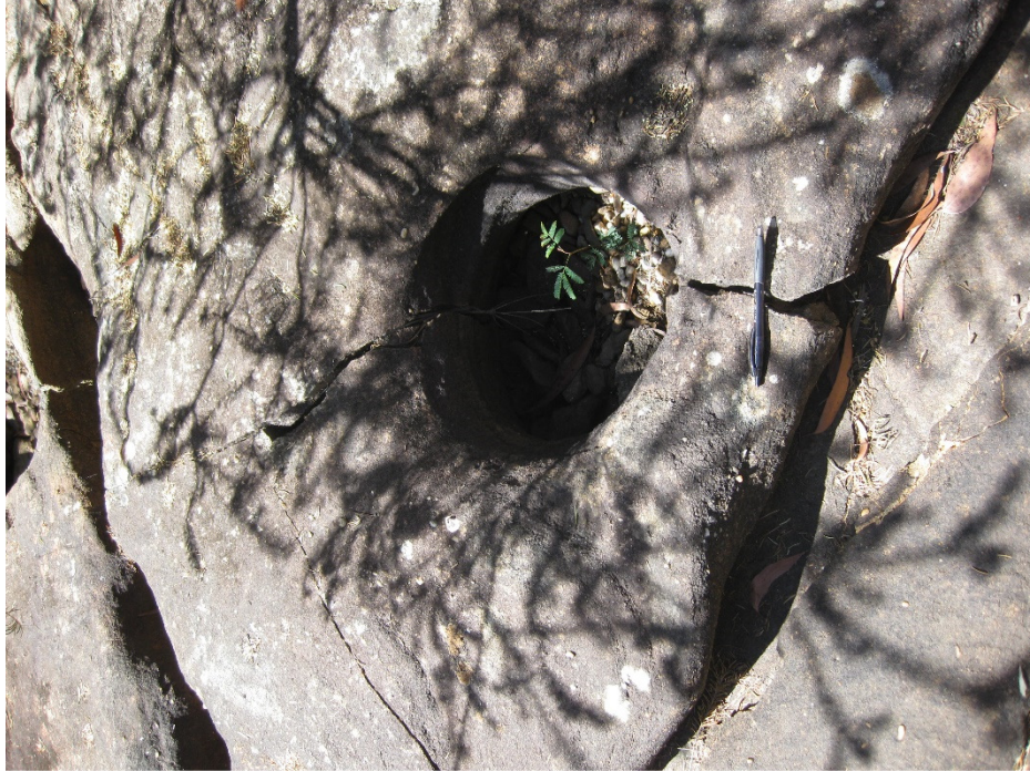
Photo 3 - Cracked and Dry Pool along 2nd Order Creek No. WC21, Area 3B (>2 years since mining of LW 10)
