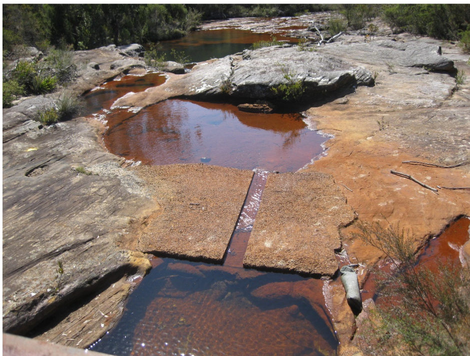
Photo 10 - Stream Gauging Weir along Sandy Creek to east of Area 3A
