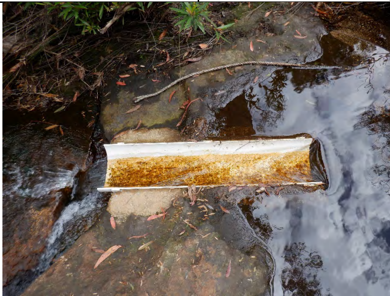
LC5S1, looking at the weir. Taken 14/4/2021.
