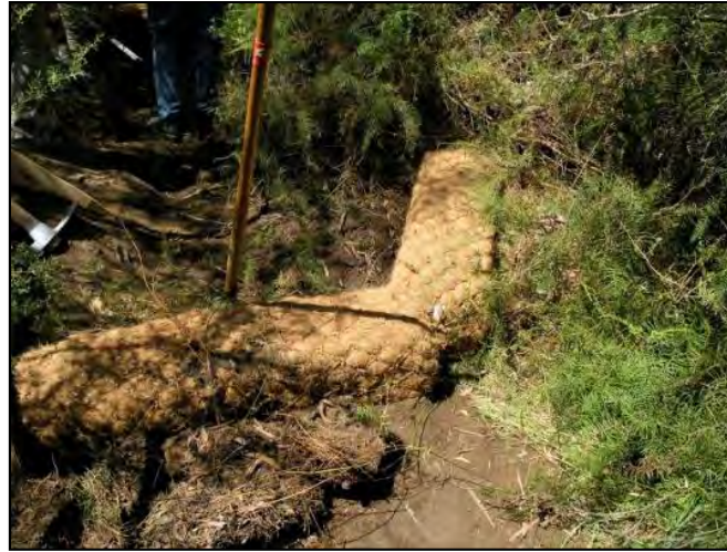
Figure 6-2 Square coir logs for knick point control
