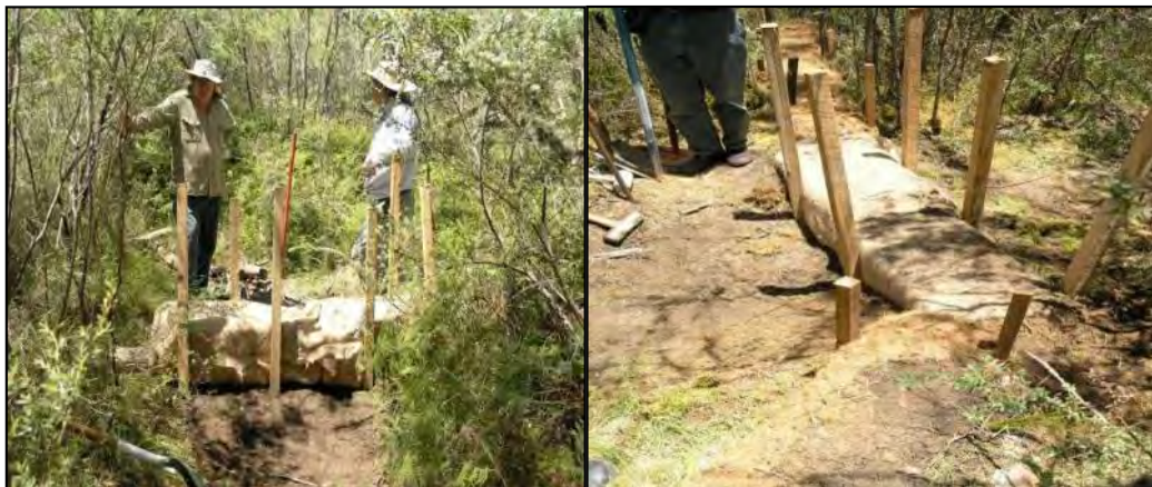
Figure 6-3 Installation of square coir logs
