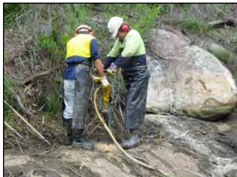
(a) Drilling into the bedrock
