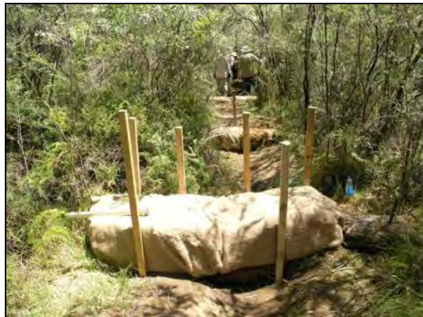
Figure 6-5 Small coir log dams with fibre matting
