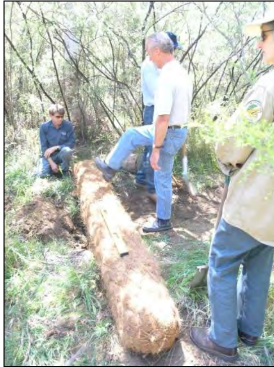
Figure 6-6 Round coir logs installed to spread water
