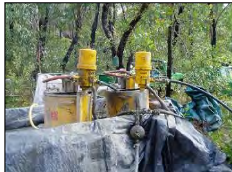
(b) Grout pump station setup
