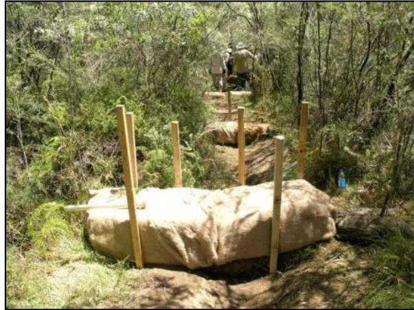
Figure 5-5 Small Coir Log Dams with Fibre Matting
