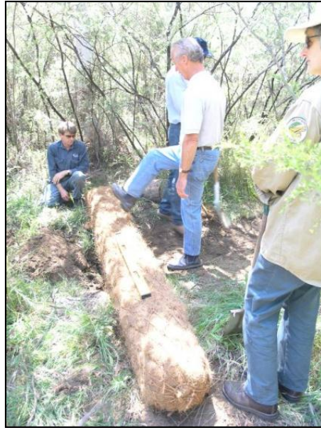
Figure 5-6 Round Coir Logs Installed to Spread Water
