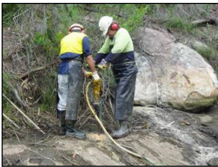
(a) Drilling into the bedrock
