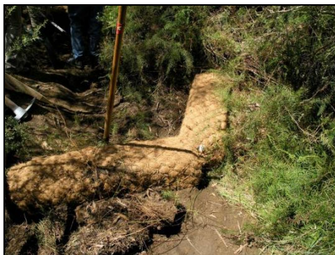
Figure 5-2 Square Coir Logs for Knick Point Control
