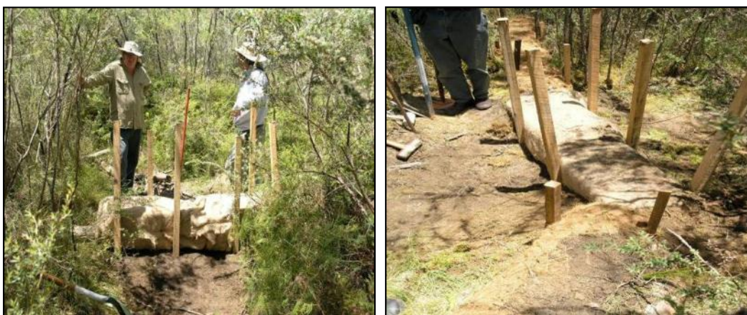
Figure 5-3 Installation of Square Coir Logs
