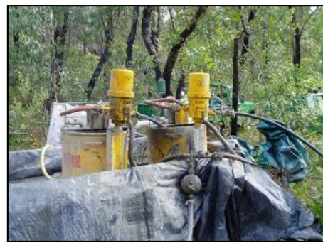
(b) Grout pump station setup
