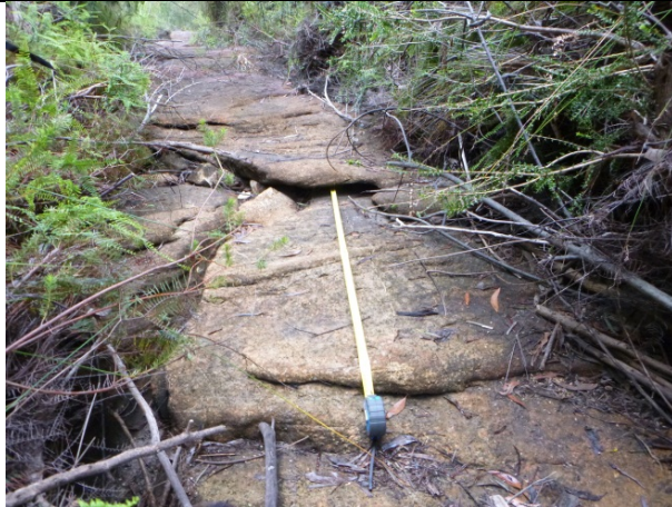
Photo 24: Impact DA3B_LW10_018. Taken on 18/12/2014
