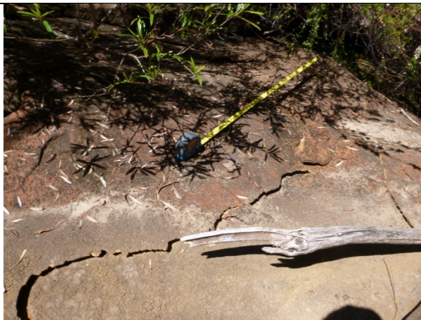
Photo 26: Impact DA3B_LW10_009. Taken on 18/11/2014
