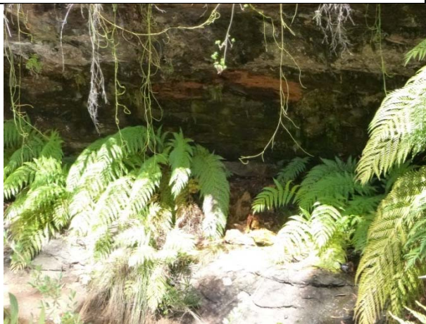
Photo 75: Impact LW9_027, small rockfall adjacent to Pool 10. Taken on 28/01/2014.
