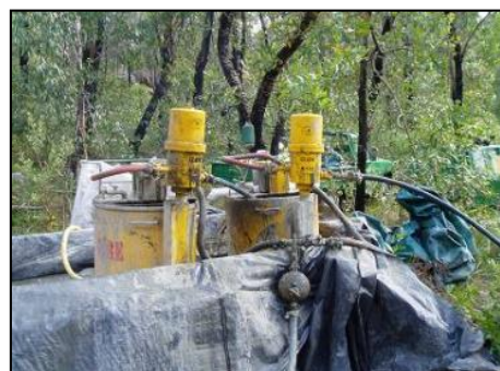
(b) Grout pump station setup
