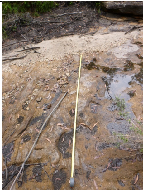
Photo 31: Impact DA3B_LW10_014-Fracture to base of WC21_Pool 23, looking across stream. Photo taken on 4/12/2014.
