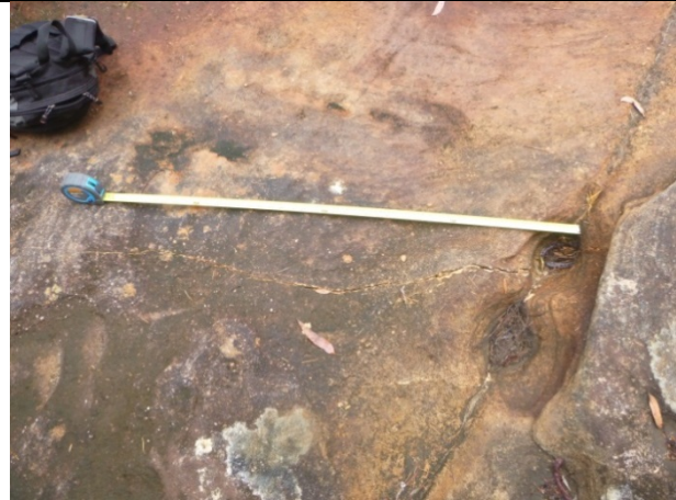
Photo 25: Impact DA3B_LW10_019. Taken on 18/12/2014
