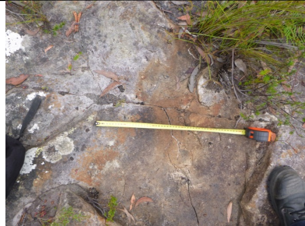
Photo 49: Impact LW9_022- Rock fracturing to Rockbar 18. Taken on 2/01/2014.
