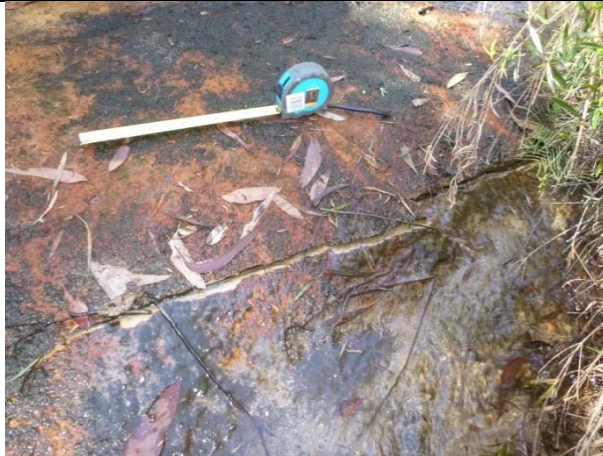
Photo 10: Impact LW10_007- Fracturing to downstream end of Rockbar 26. Taken on 18/11/2014.
