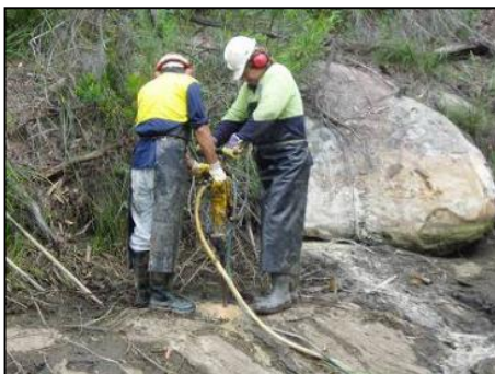
(a) Drilling into the bedrock
