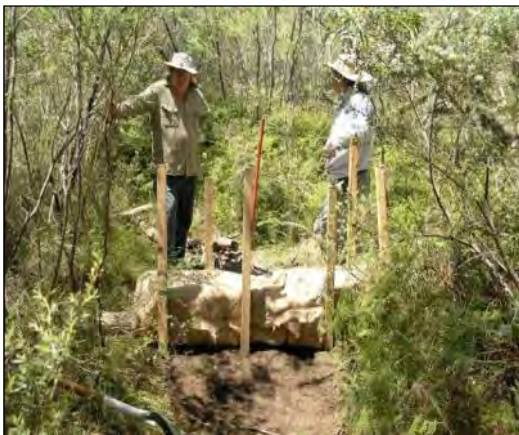
Figure 5-3 Installation of Square Coir Logs
