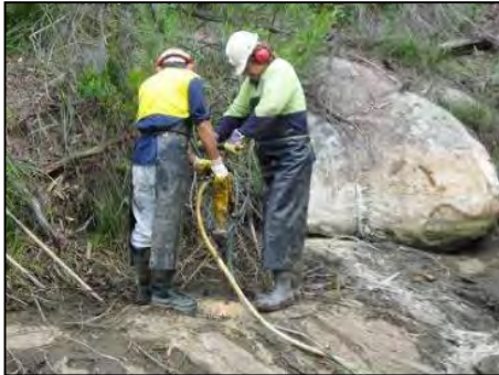
(a) Drilling into the bedrock
