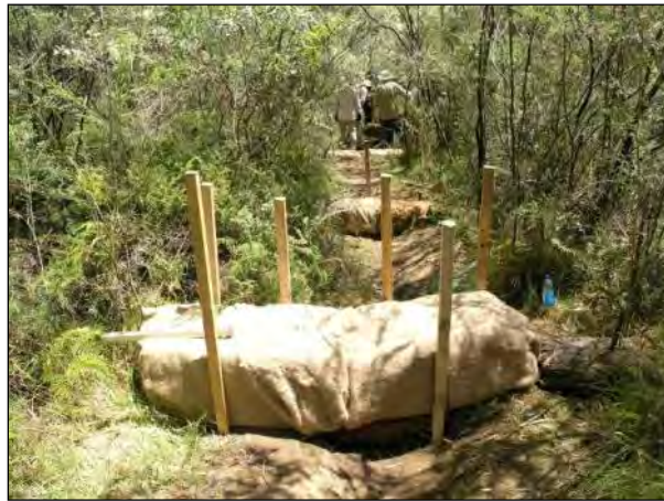
Figure 5-5 Small Coir Log Dams with Fibre Matting
