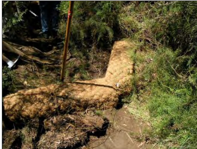
Figure 5-2 Square Coir Logs for Knick Point Control
