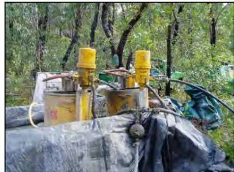
(b) Grout pump station setup
