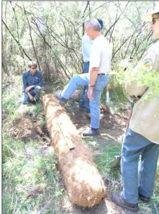
Figure 5-6 Round Coir Logs Installed to Spread Water
