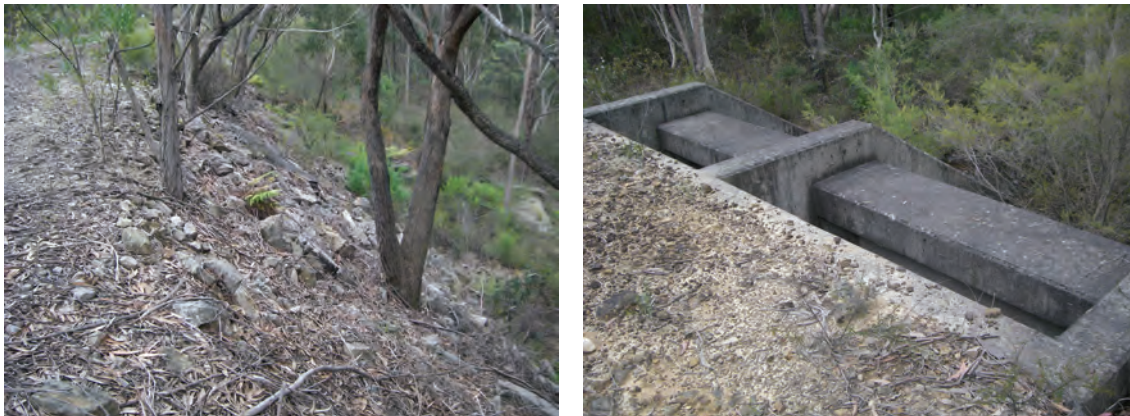
Fig. 6.2 Photographs of an Embankment and Drainage Culvert
