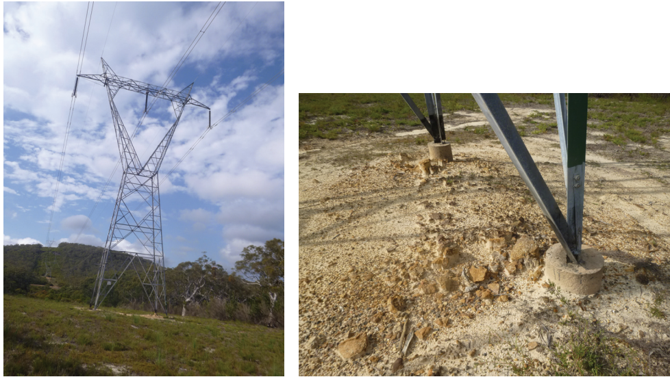
Fig. 6.3 330 kV transmission tower
