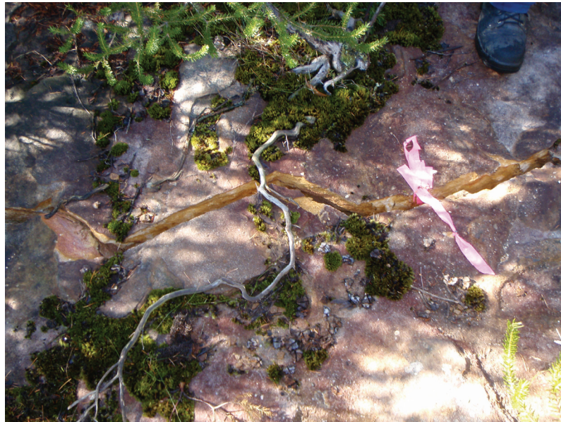
Fig. 5.16 Fracturing in the rockbar downstream of Swamp Den01 (Source: IC)
