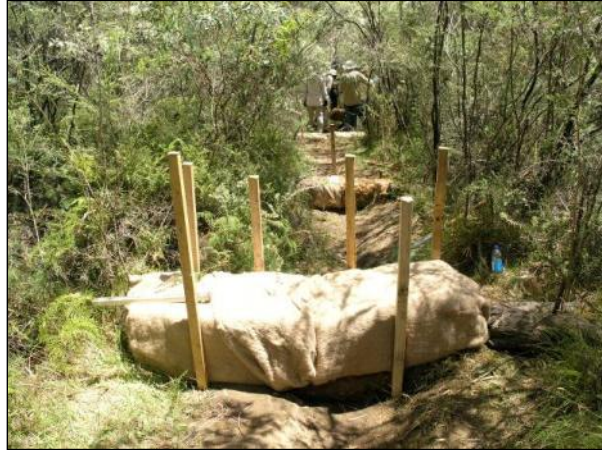
Figure 6-5 Small Coir Log Dams with Fibre Matting
