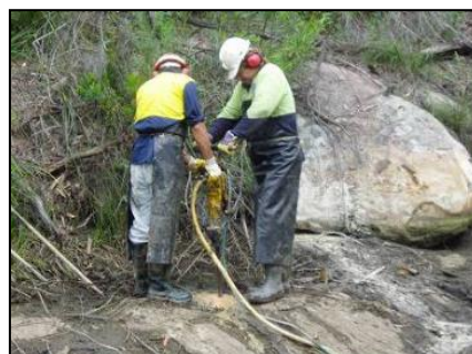
(b) Grout pump station setup
