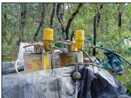
(a) Drilling into the bedrock
