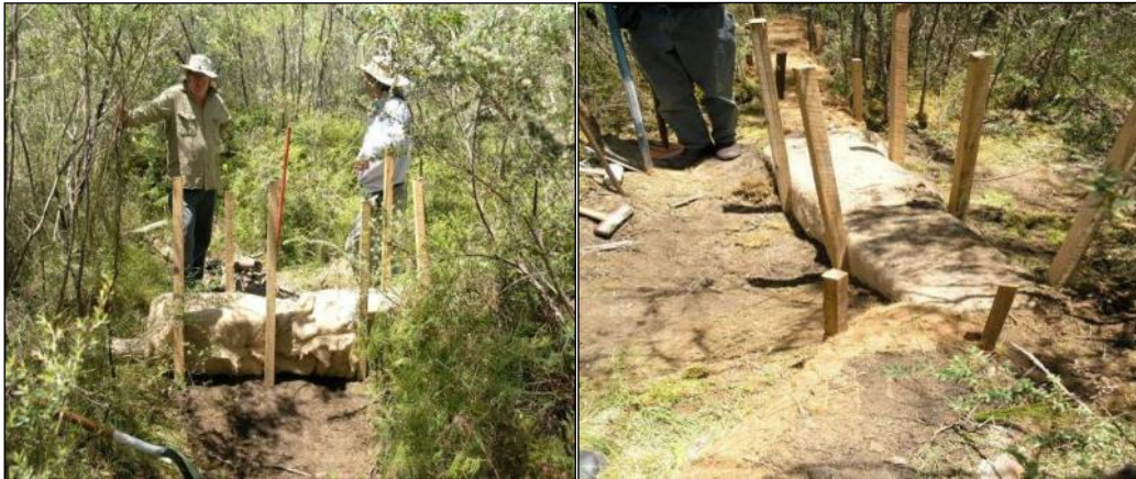
Figure 6-3 Installation of Square Coir Logs
