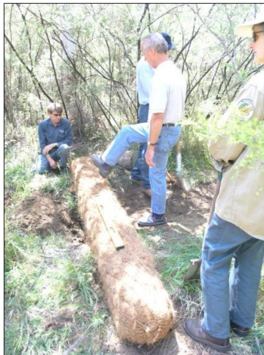
Figure 6-6 Round Coir Logs Installed to Spread Water
