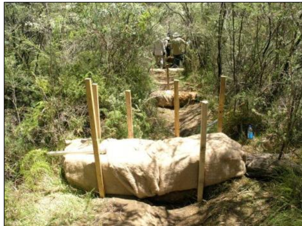
Figure 6-5 Small Coir Log Dams with Fibre Matting
