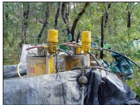
(b) Grout pump station setup
