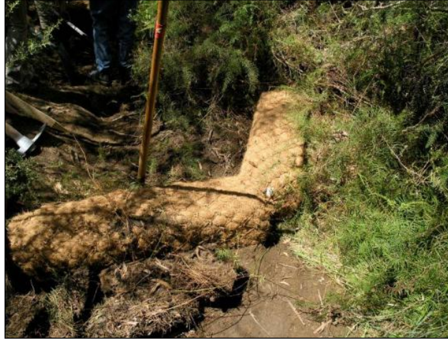
Figure 6-2 Square Coir Logs for Knick Point Control
