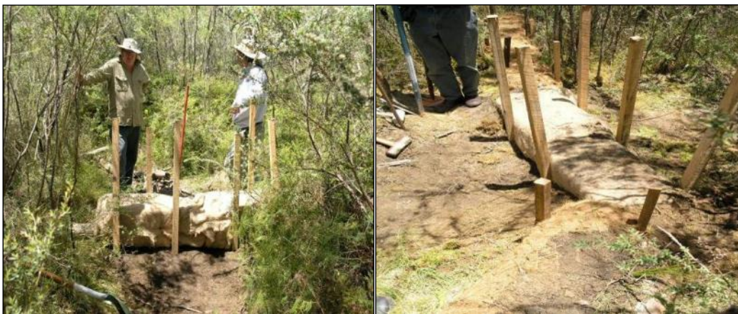
Figure 6-3 Installation of Square Coir Logs
