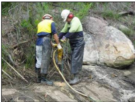
(a) Drilling into the bedrock
