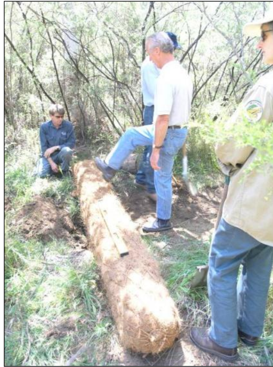
Figure 6-6 Round Coir Logs Installed to Spread Water
