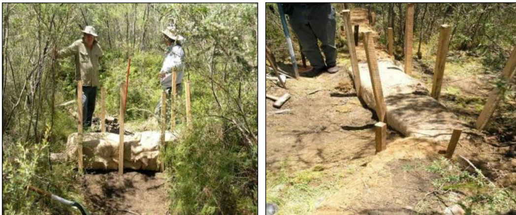
Figure 5-3 Installation of Square Coir Logs
