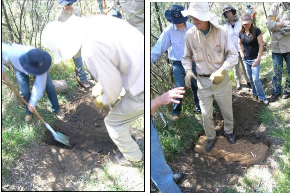
Figure 5-4 Trenching and Positioning of the First Layer of Coir Logs and Construction of a Small Dam in a Channel
