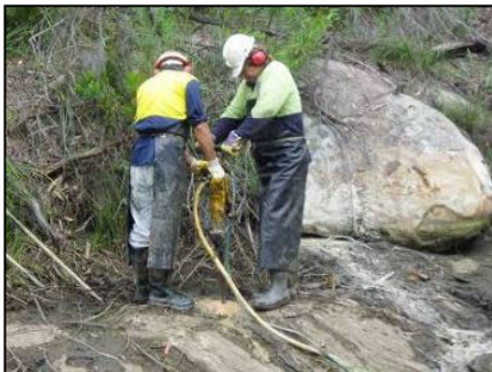
(a) Drilling into the bedrock
