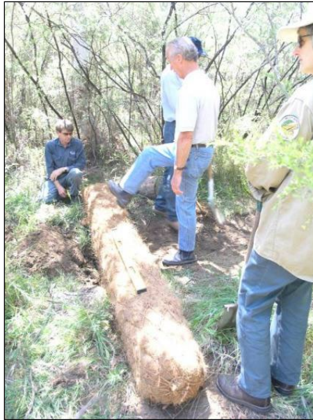
Figure 5-6 Round Coir Logs Installed to Spread Water
