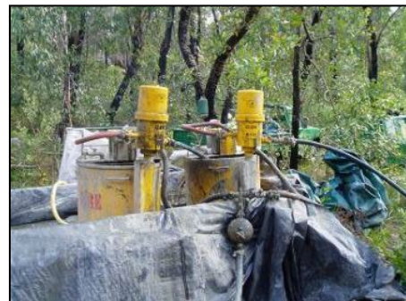
(b) Grout pump station setup
