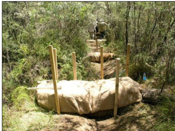
Figure 5-5 Small Coir Log Dams with Fibre Matting
