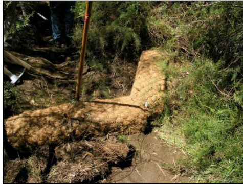
Figure 5-2 Square Coir Logs for Knick Point Control
