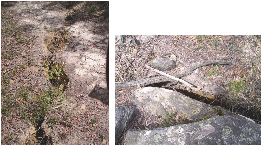
Fig. 5.11 Surface tension cracking due to downslope movements at Dendrobium Mine
