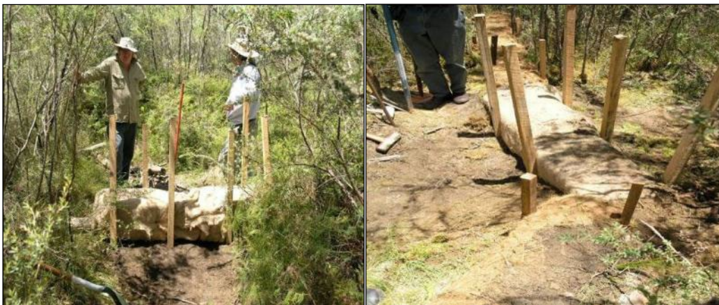
Figure 6-3 Installation of Square Coir Logs
