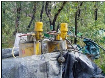
(a) Drilling into the bedrock
