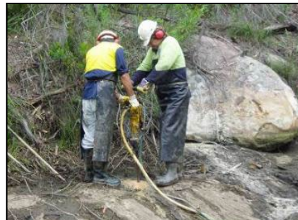
(b) Grout pump station setup
