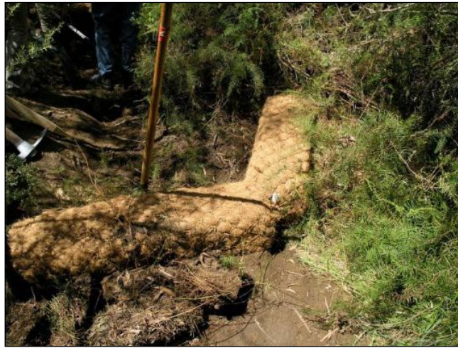
Figure 6-2 Square Coir Logs For Knick Point Control
