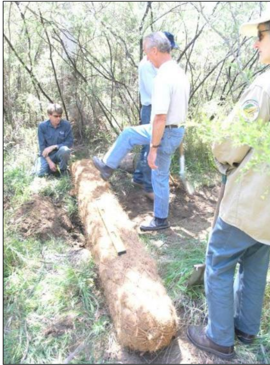
Figure 6-6 Round Coir Logs Installed to Spread Water
