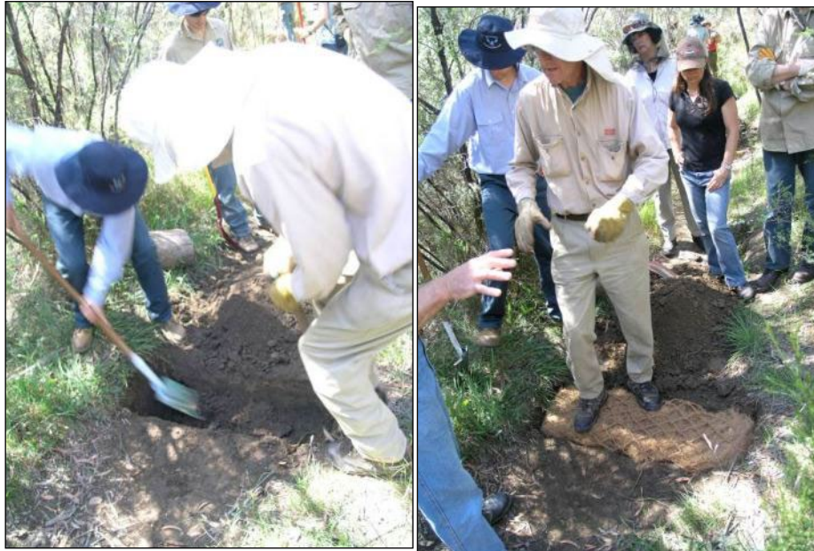
Figure 6-4 Trenching & Positioning of the First Layer of Coir Logs and Construction of a Small Dam in an Eroding Swamp Channel
