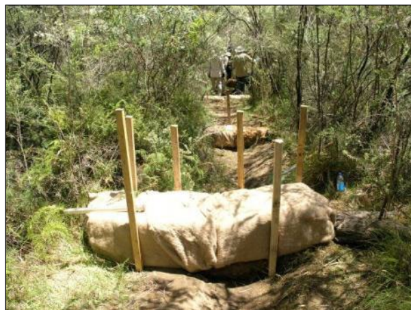
Figure 6-5 Small Coir Log Dams with Fibre Matting
