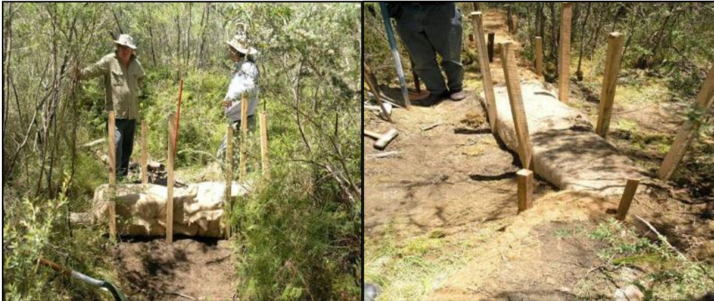
Figure 6-3 Installation of Square Coir Logs
