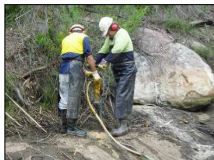
(b) Grout pump station setup
