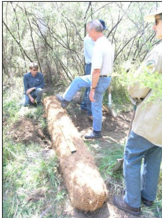
Figure 6-6 Round Coir Logs Installed to Spread Water
