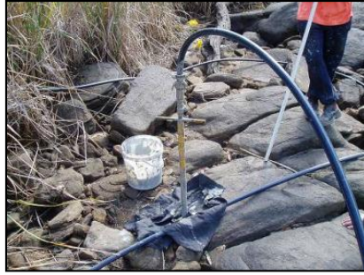
(c) Injecting grout into bedrock via a specially designed packer system
