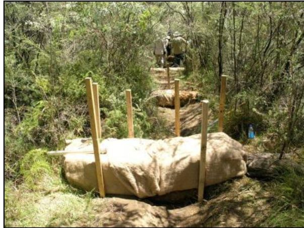
Figure 6-5 Small Coir Log Dams with Fibre Matting
