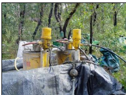
(a) Drilling into the bedrock
