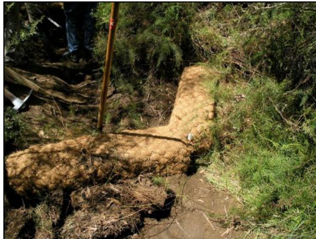
Figure 6-2 Square Coir Logs For Knick Point Control
