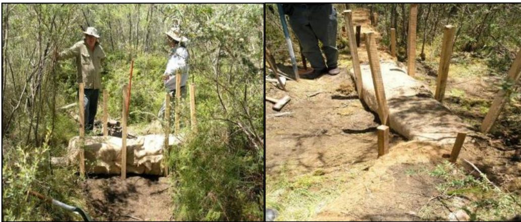
Figure 6-3 Installation of Square Coir Logs
