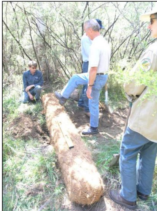
Figure 6-6 Round Coir Logs Installed to Spread Water
