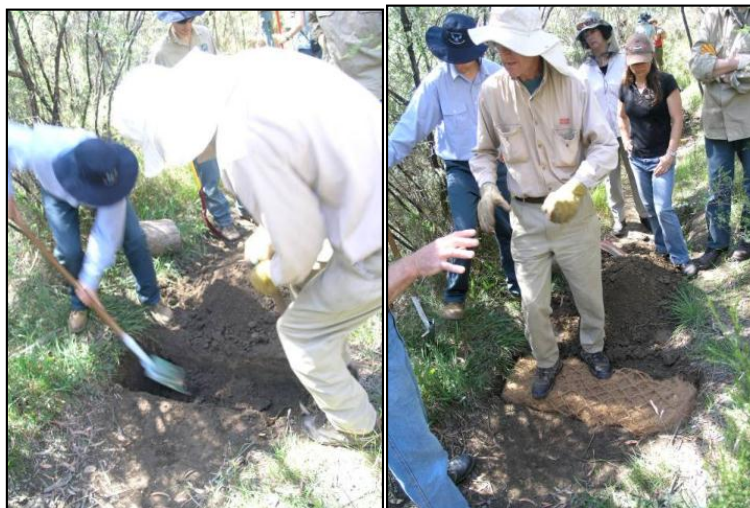
Figure 6-4 Trenching and Positioning of the First Layer of Coir Logs and Construction of a Small Dam in a Channel
