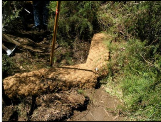
Figure 6-2 Square Coir Logs for Knick Point Control
