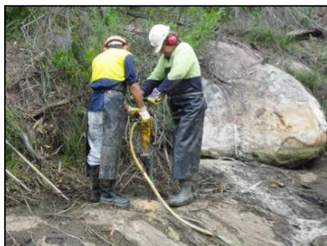
(a) Drilling into the bedrock
