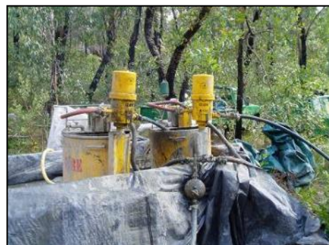
(b) Grout pump station setup
