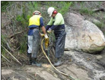
(a) Drilling into the bedrock
