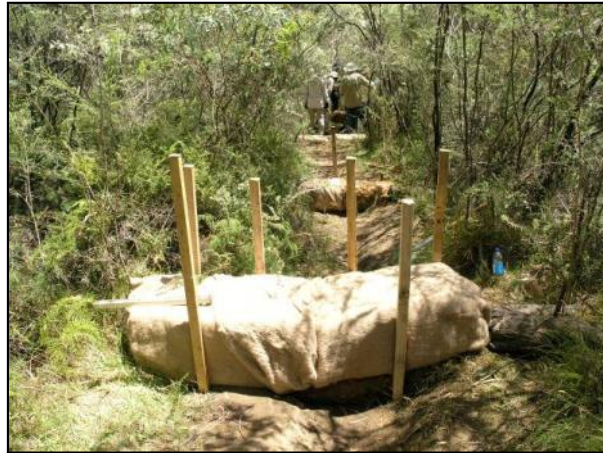
Figure 5-5 Small Coir Log Dams with Fibre Matting
