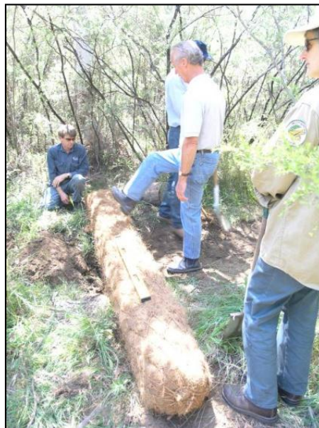
Figure 5-6 Round Coir Logs Installed to Spread Water
