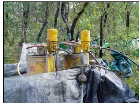
(b) Grout pump station setup
