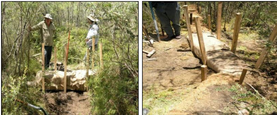
Figure 5-3 Installation of Square Coir Logs
