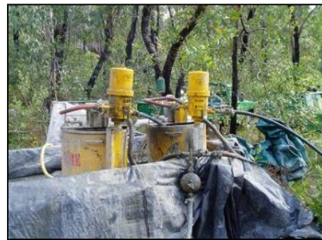
(b) Grout pump station setup
