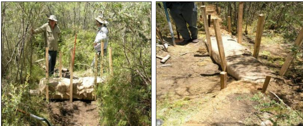
Figure 5-3 Installation of Square Coir Logs
