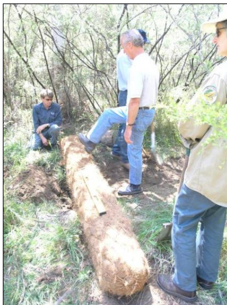
Figure 5-6 Round Coir Logs Installed to Spread Water
