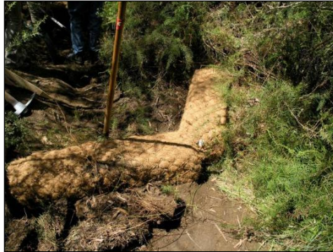
Figure 5-2 Square Coir Logs for Knick Point Control
