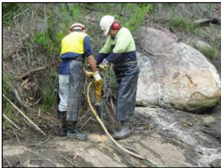
(a) Drilling into the bedrock
