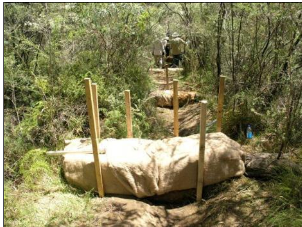
Figure 5-5 Small Coir Log Dams with Fibre Matting
