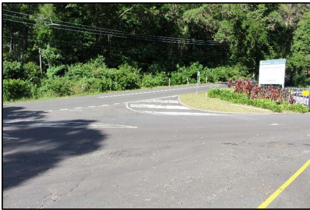
Plate 1: Entrance to Dendrobium mine from Cordeaux road at the western end of the substation. South east aspect. (Source: Niche 2018).
