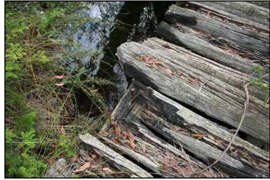
Plate 7: Decking elements, square sawn or “pencil” ends.
