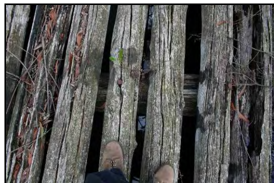
Plate 4: Timber corduroy bridge across tributary of Cordeaux River. Plate 5: Circular section deck timbers.
