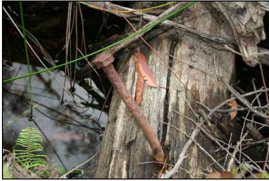
Plate 6: Iron bolts used to fix deck timbers to bearers.
