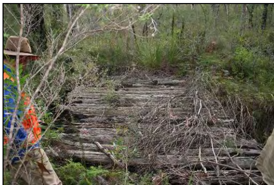
Plate 4: Timber corduroy bridge across tributary of Cordeaux River. Plate 5: Circular section deck timbers.
