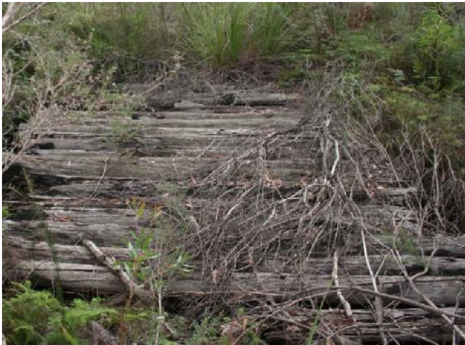
Fig. 2.7 Historic Bridge in Area 3C
