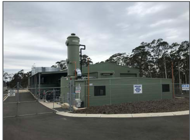
Figure 2: Water Filtration Plant Expansion - Main processing facility.
