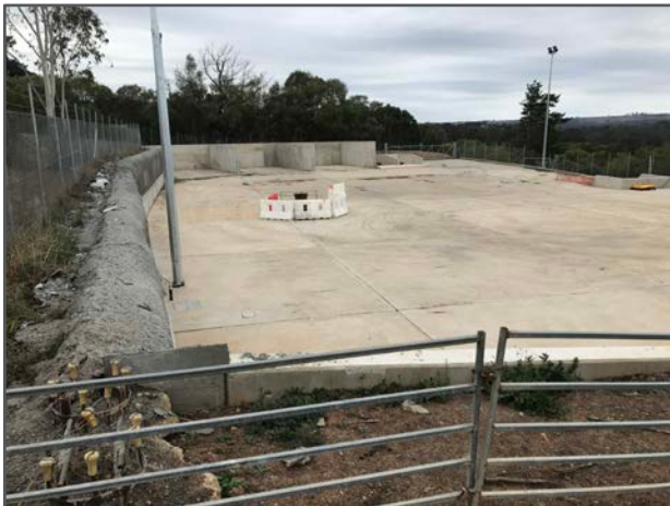
Figure 1: Concrete pad construction at the Vent Shaft 6 site concrete/ballast borehole.
