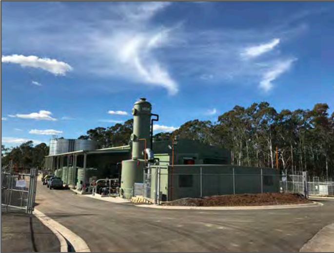
Figure 2: Water Filtration Plant Expansion - Main processing facility
