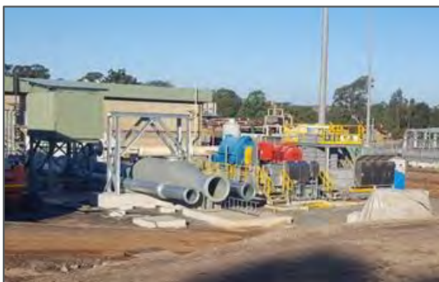
Figure 4: Construction progress of gas drainage plant at Appin East
