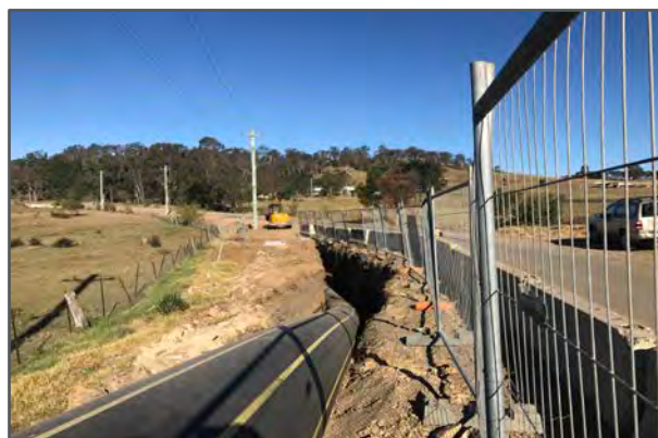
Figure 5: Buried gas pipeline along Brooks Point Road
