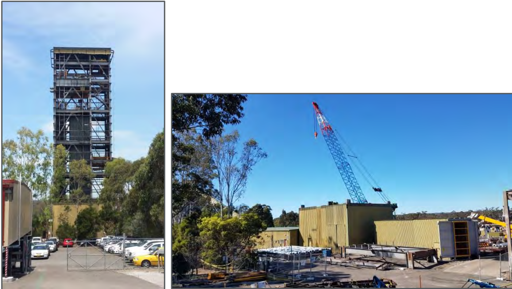
Figure 13: Demolition of the bulk coal winder building
