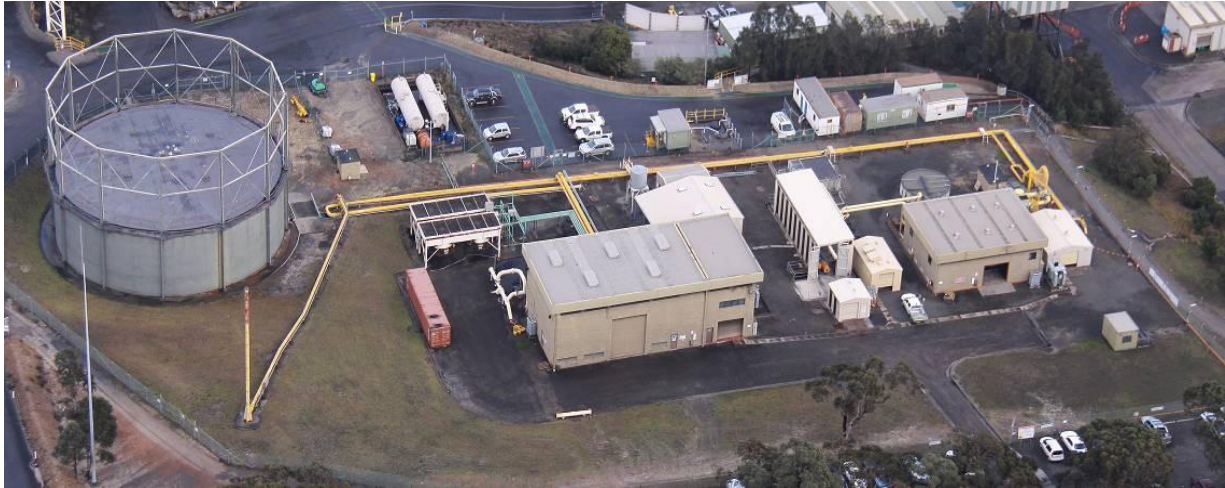
Figure 14: Methane extraction plant – West Cliff
