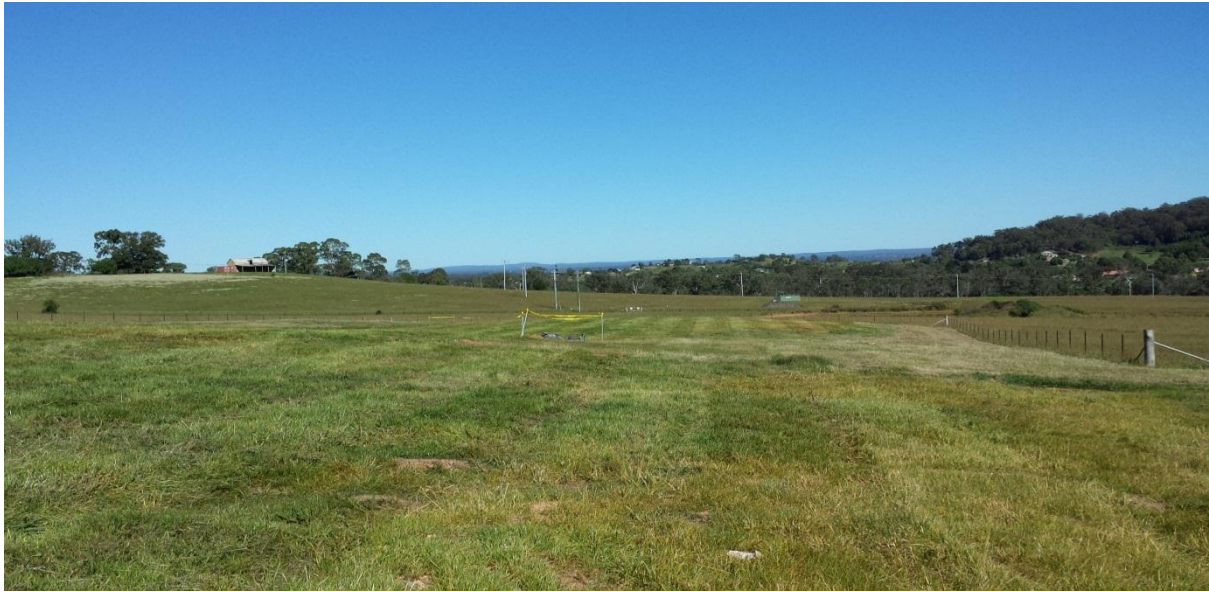
Figure 12: LW 704 pads during rehabilitation works
