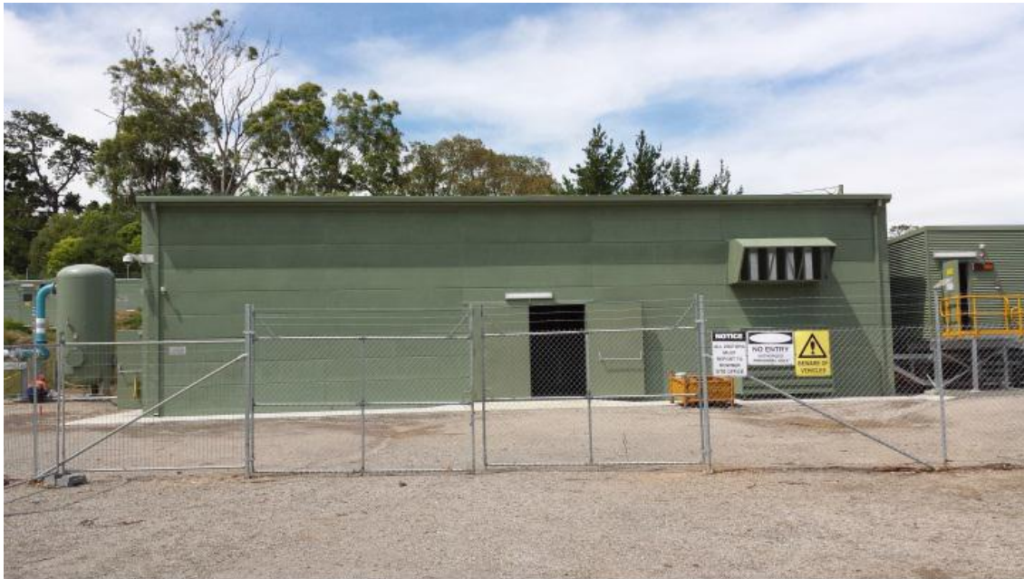
Figure 2: VS#6 Air Compressor Shed.
