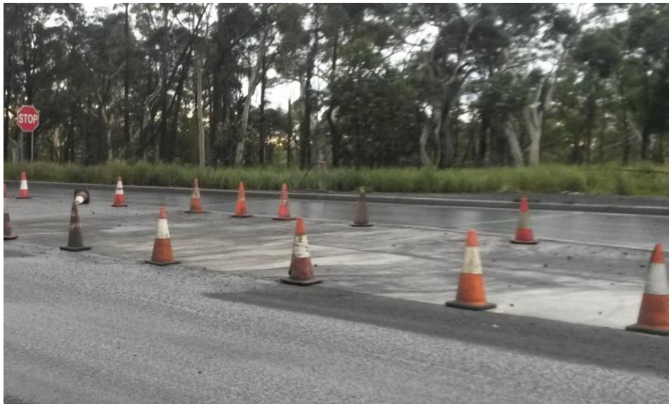
Figure 4: New concrete section of road at truck turn-out area.
