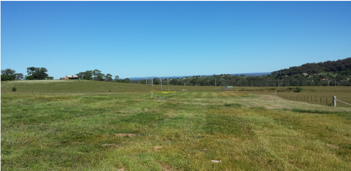
Figure 12: LW 704 pads during rehabilitation works
