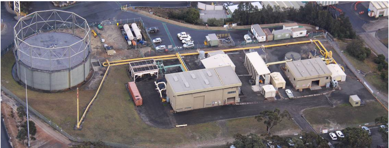
Figure 14: Methane extraction plant – West Cliff
