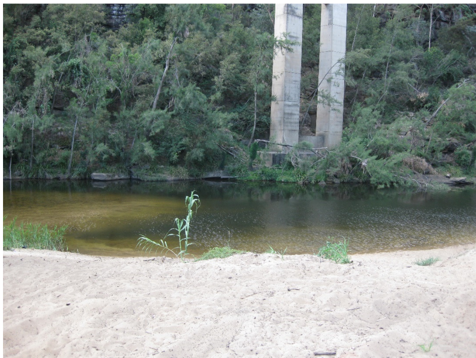
Photo 10 - Nepean River at Hume Highway Bridge Crossing - Area 9
