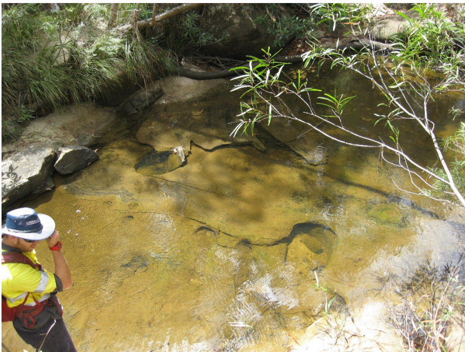
Photo 2 - Cracking to rock bar along Georges River - Level 1 Impact (no water diversion)
