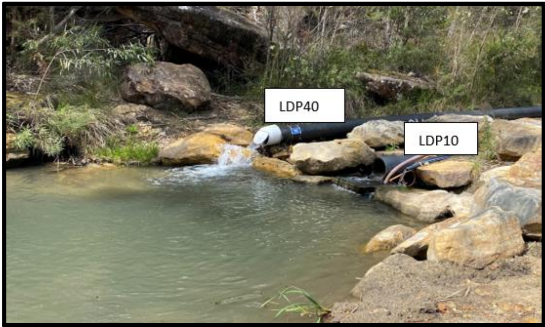
Figure 2. LDP10 and LDP40 discharge pipes flowing into Point 10 site at Brennans Creek.
