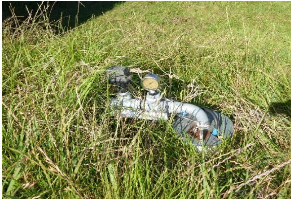
Photo 1 Borehole GW110671, taken on 15 November 2017 during pre-mining inspection.
