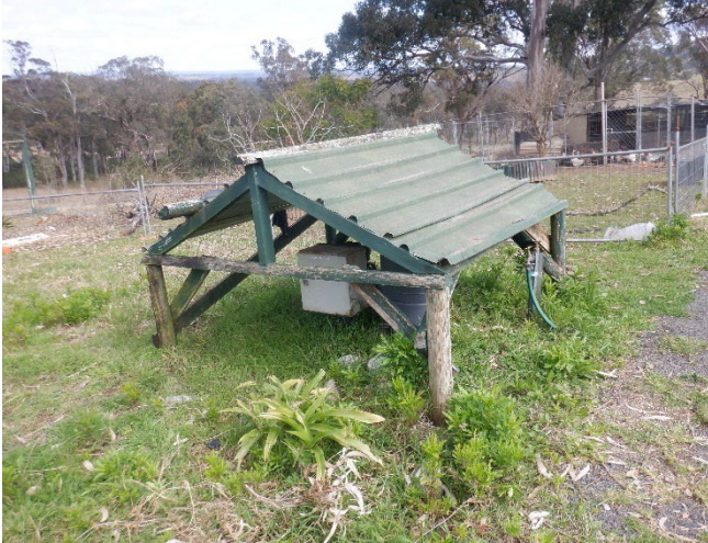
Photo 7: Borehole GW072249 and cover. Taken on 26 August 2022.
