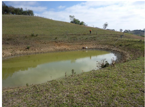
Photo 8: Property dam. Taken on 14/09/2018
