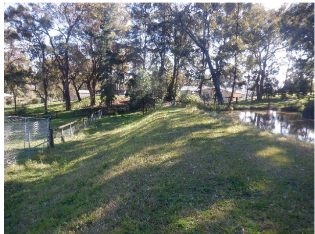
Photo 10: Dam Wall. Taken at 010 degrees on 5 September 2022.
