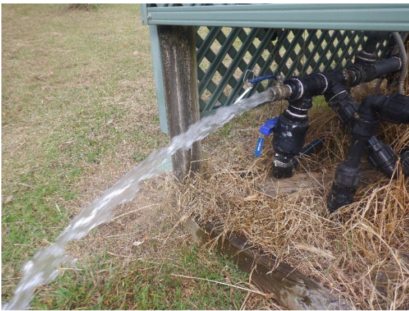
Photo 15: GW105534 discharge, new sample point direct from bore. Taken on 20 April 2023
