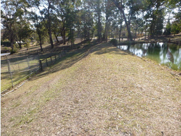
Photo 7: Dam Wall. Taken at 010 degrees on 23 August 2017.
