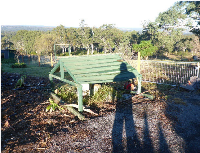
Photo 5: Borehole GW072249. Taken on 6 June 2019.
