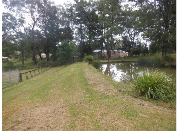
Photo 14: Dam Wall. Taken at 010 degrees on 20 April 2023.
