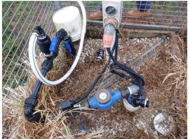
Photo 16: New pump installed for the borehole. Taken 5 October 2022.
