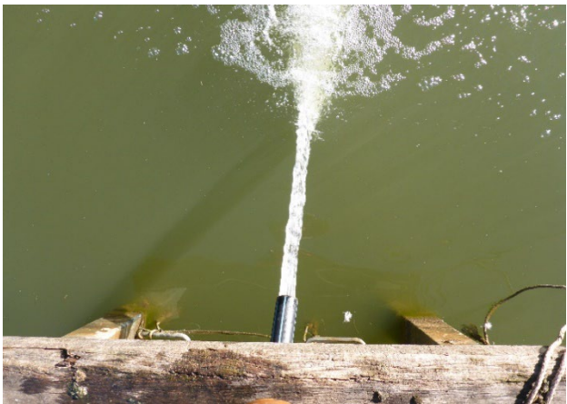
Photo 5: Borehole outlet into Dam 1. Taken on 6 June 2019.
