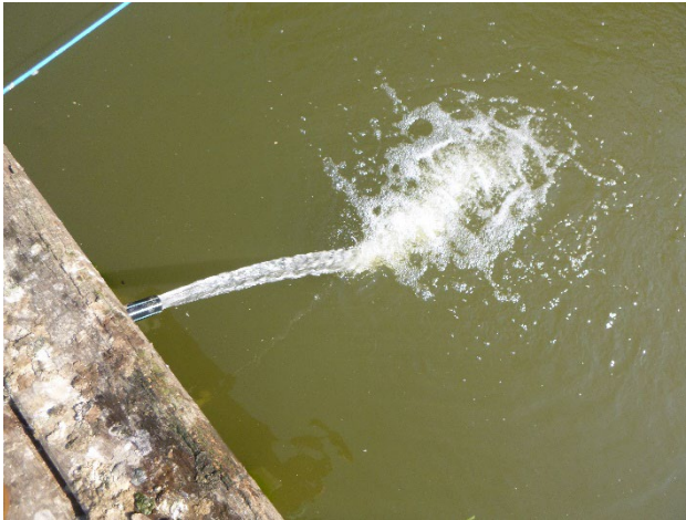
Photo 9: Borehole outlet into Dam 1. Taken on 29 April 2021
