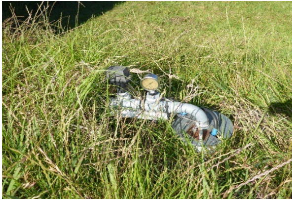
Photo 1: Borehole GW110671, taken on 15 November 2017 during pre-mining inspection.
