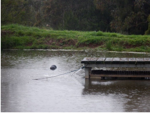
Photo 13: Borehole outlet into Dam 1. Taken on 5 October 2022.
