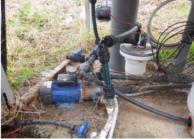
Photo 7: The capped borehole GW100673. Photo taken on 26 August 2022.
