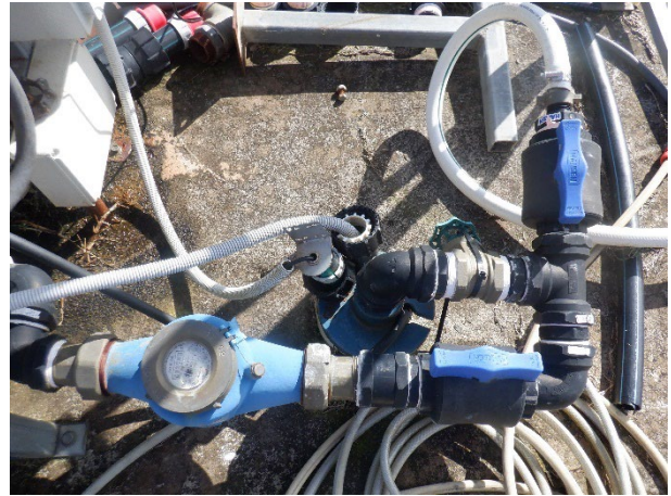
Photo 8: Closeup of borehole GW104602 and pump. Taken on 26 August 2022.
