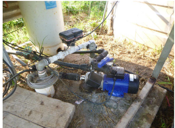
Photo 4: The capped borehole GW100673. Photo taken on 29 April 2021.
