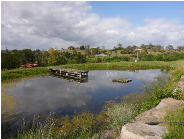
Photo 3: Dam 1. Taken on 2 November 2017.
