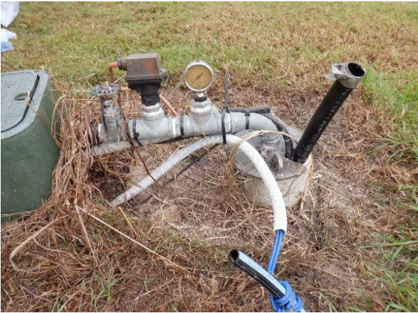
Photo 5: Borehole GW110671, taken on 25 May 2021 during post-mining inspection.
