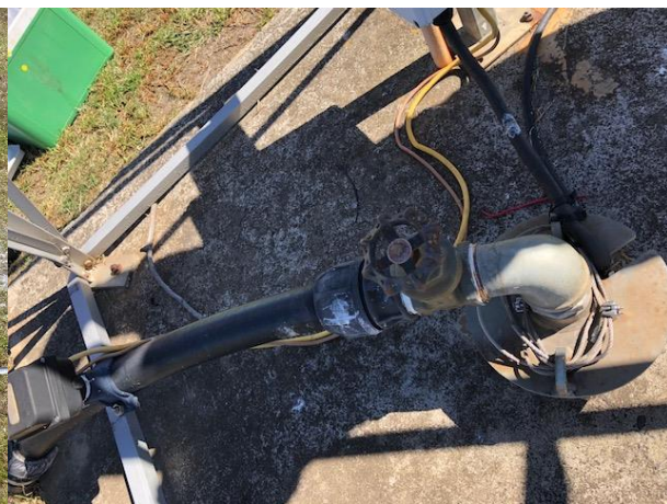
Photo 2: Closeup of borehole GW104602. Taken on 16 April 2018.
