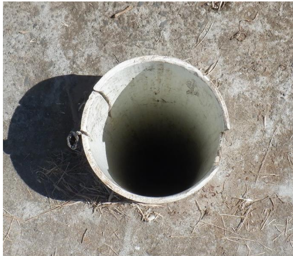
Photo 5: Closeup of borehole GW104602. Taken on 3 May 2021.
