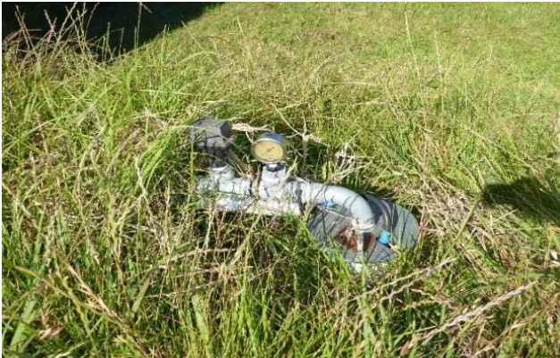
Photo 1: Borehole GW110671, taken on 15 November 2017 during pre-mining inspection.
