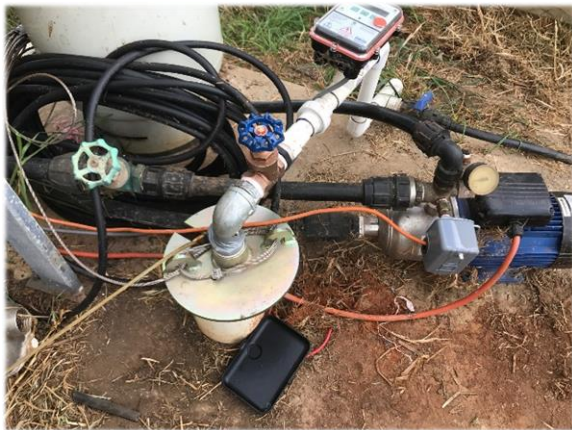
Photo 1: The capped borehole GW100673. Taken 16 May 2018.
