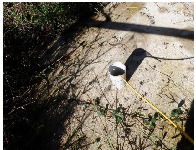
Photo 4: Looking at the borehole, with new collar. Taken on 10 May 2021.
