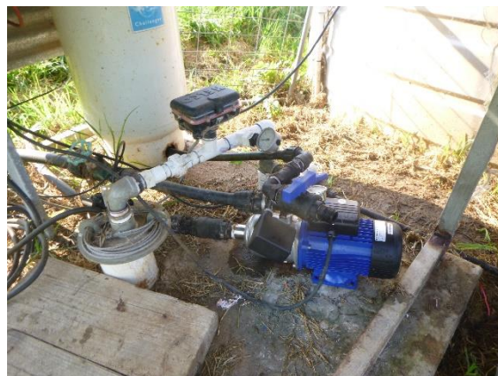
Photo 4: The capped borehole GW100673. Taken 29 April 2021.
