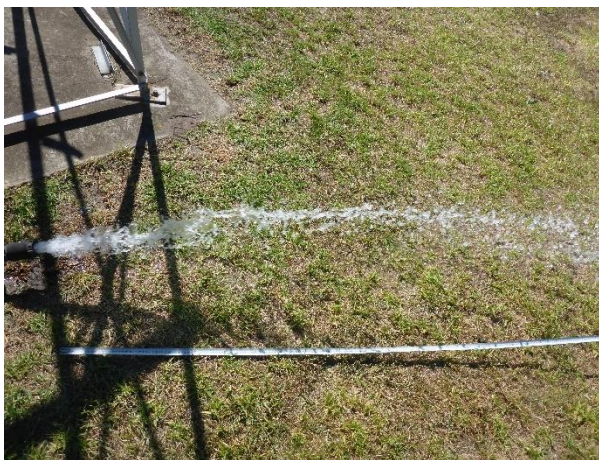
Photo 1: Water pressure from pump. Taken on 16 April 2018.
