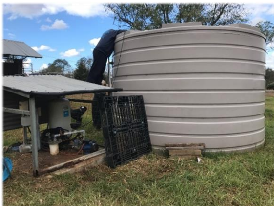
Photo 3: Settling tank where water from GW100673 is pumped. Taken 16 May 2018.
