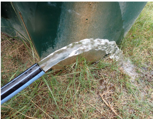
Photo 5: Borehole GW101986 outflow. Taken on 28/09/2023.
