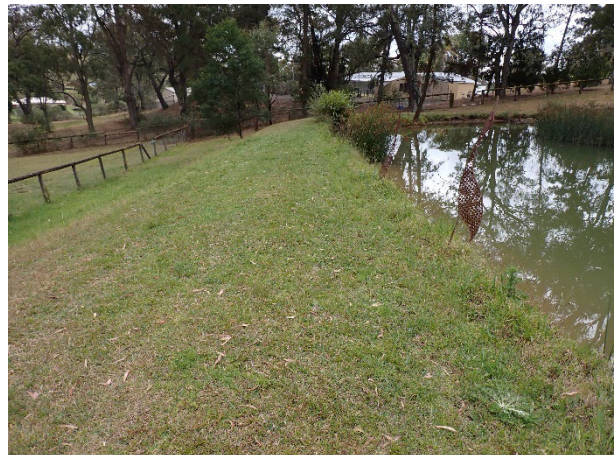
Photo 10: Dam Wall. Taken at 010 degrees on 28 September 2023.
