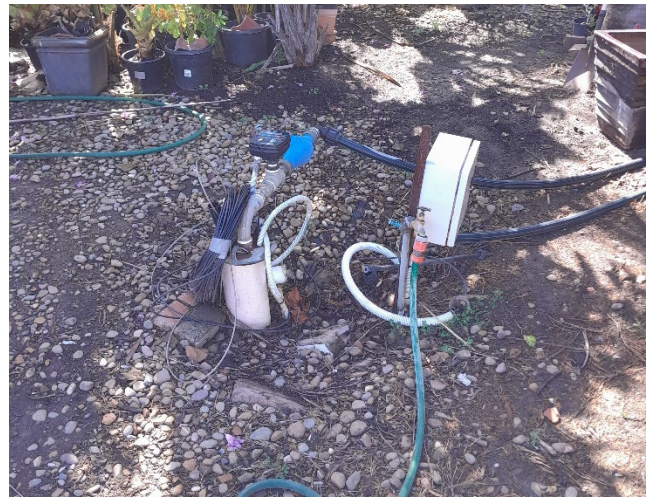
Photo 2: Borehole during post-mining inspection. Taken on 28/09/2023
