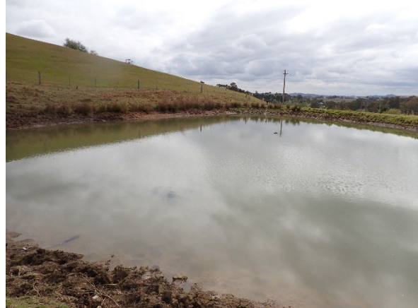
Photo 10: Property dam. Taken on 28/09/2023
