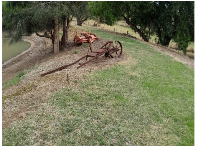
Photo 10: Dam wall during post-mining inspection, looking west. Taken on 28/09/2023
