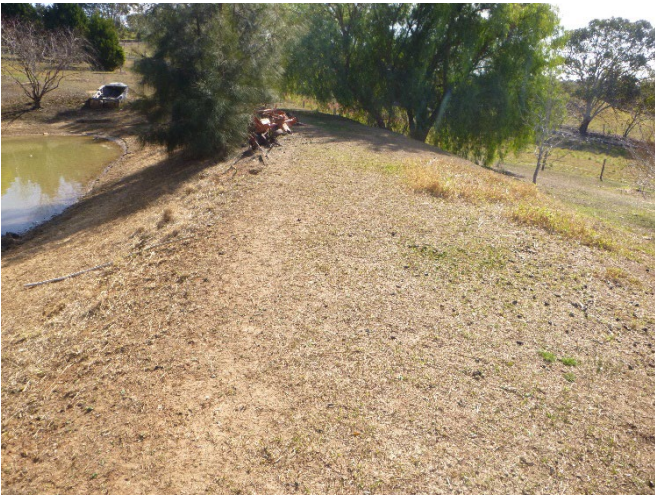
Photo 9: Dam wall during initial post-mining inspection, looking west. Taken on 25/7/2018
