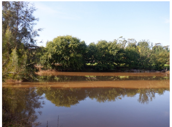
Photo 6: Soil cracking no longer visible due to high water level in dam, looking south. Taken on 17/03/2022
