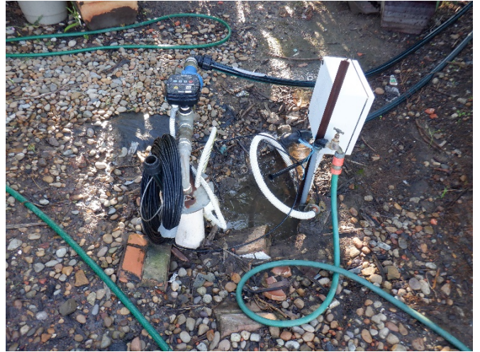
Photo 2: Borehole during post-mining inspection. Taken on 17/03/2022
