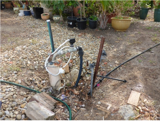
Photo 1: Borehole GW105376. Taken on 19/02/2018.
