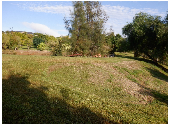
Photo 10: Dam wall during post-mining inspection, looking northwest. Taken on 17/03/2022
