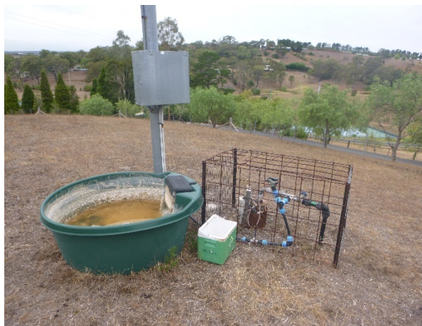
Photo 1: Photo of GW101986 and pump. Taken 22/2/2018.
