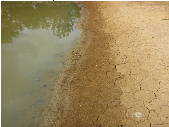
Photo 5: Soil cracking present around extent of dam edges observed during pre-mining inspection. Taken on 19/02/2018.
