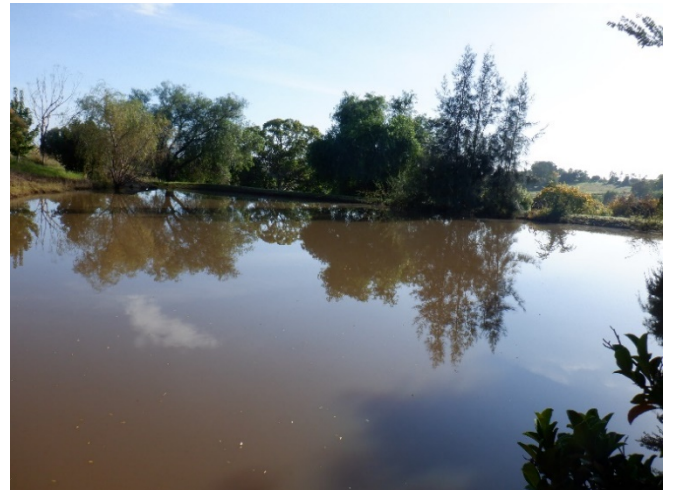
Photo 4: Dam during post-mining inspection. Taken on 17/03/2022
