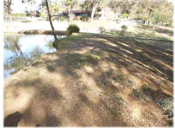
Photo 8: Image of Dam Wall. Taken at 260 degrees on the 25 th July 2018.
