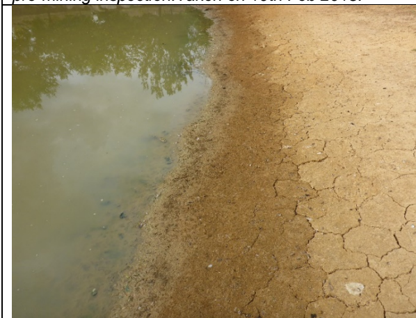
Photo 5: Soil cracking present around extent of dam edges observed during pre-mining inspection. Taken on 19 th Feb 2018.
