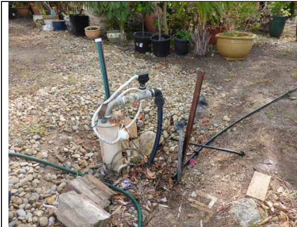
Photo 1: Borehole GW105376 location. Taken on 19 th Feb 2018.
