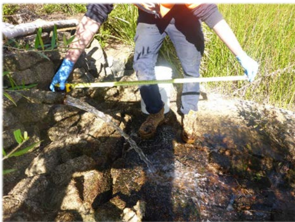
Photo 3: GW105534 outlet discharge. Taken 23 rd Aug 2017.
