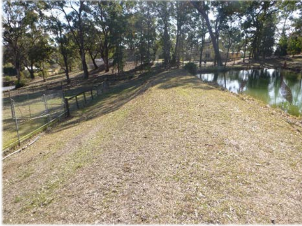
Photo 7: Image of Dam Wall. Taken at 010 degrees on the 23 rd Aug 2017.
