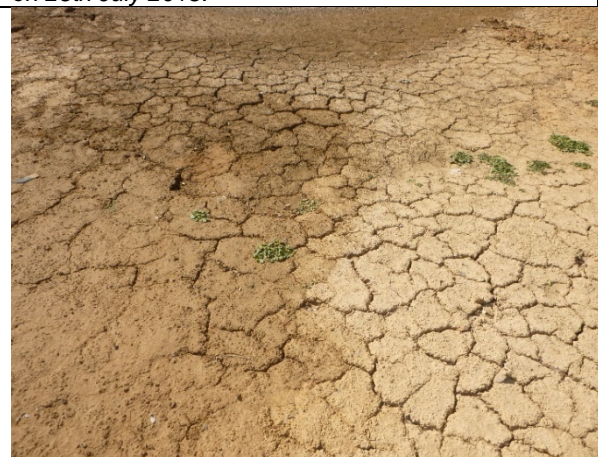
Photo 6: Soil cracking observed around dam during post-mining inspection. Taken 25 th July 2018.
