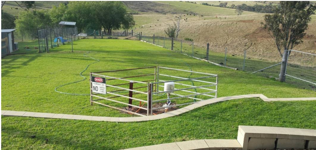
Photo 1: Temporary fencing to existing borehole
