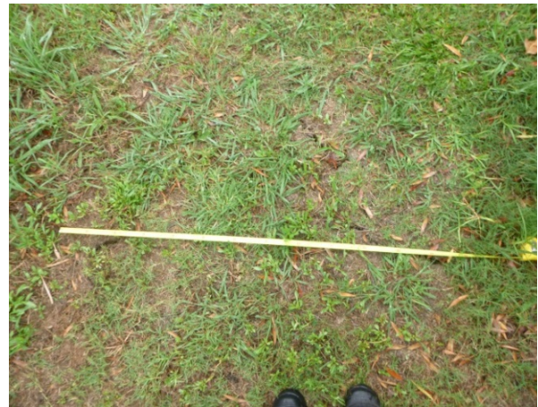
Photo 7: AA7_LW706_004; crack to base of dam wall. Taken on 04/01/2016.
