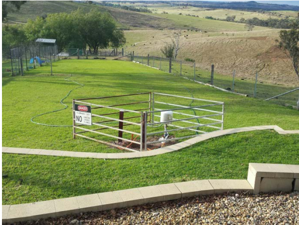
Photo 4: AA7_LW706_002; Borehole. Taken on 15/07/2015
