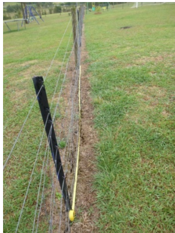
Photo 6: AA7_LW706_003; cracking along fence line. Taken on 04/01/2016.
