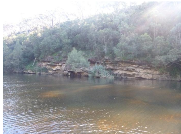
Photo 15: Cliffline downstream of site Pump 2 – NRL before mining. Taken on 30/04/14 (after start of Longwall 705).
