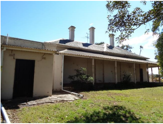
Plate 9: Main House. South elevation showing the wrap-around verandah.
