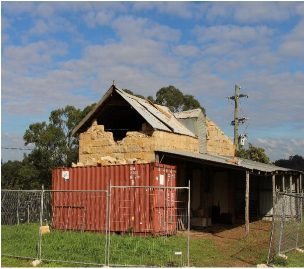
Plate 5. North western view of Mountbatten Chapel
