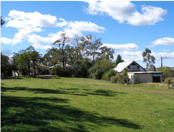
Plate 18: Exterior view showing the Main House (left) and the Cottage (right), looking west.
