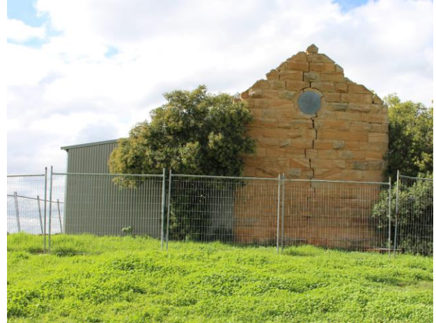
Plate 8. View of eastern wall.
