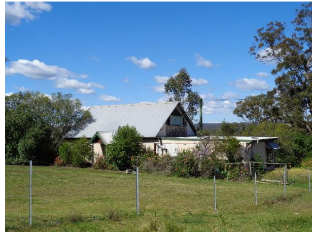
Plate 19: Cottage Building. North elevation.
