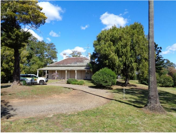
Plate 7: Main House. External view showing the entrance drive
