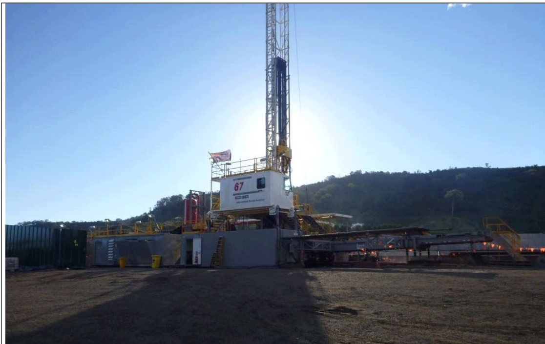
Plate 2: MSGD Borehole Drilling
