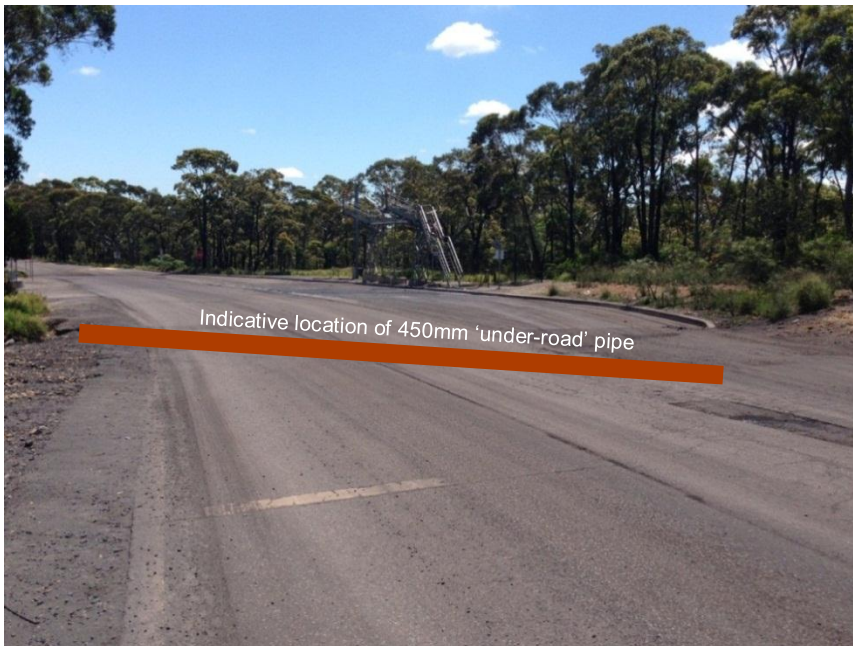
Figure 16: Indicative Location – sub-surface drainage pipe
