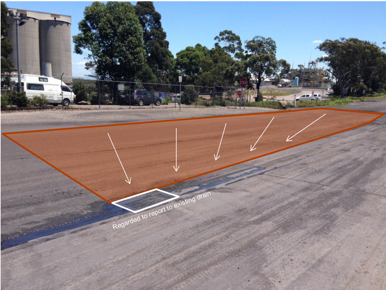
Figure 17: Area of Road Resurfacing – Northern end of Truck Tarping Area
