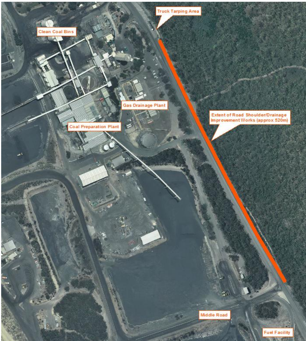
Figure 19: Extent of Road Shoulder and Drainage Improvements
